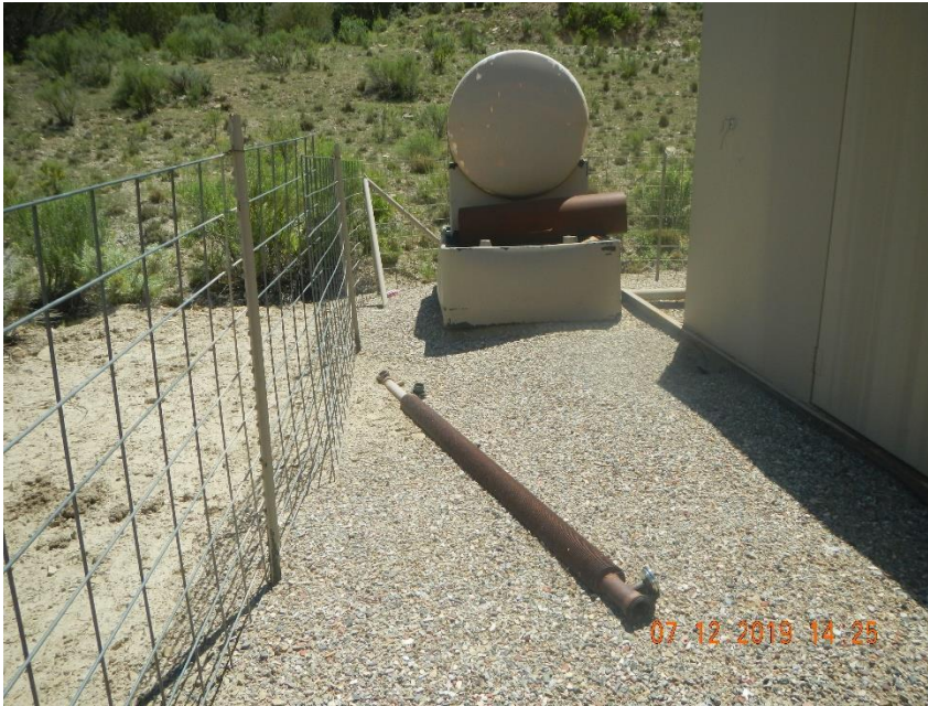
Unused equipment. Unused container and flow line for dehydrator.
