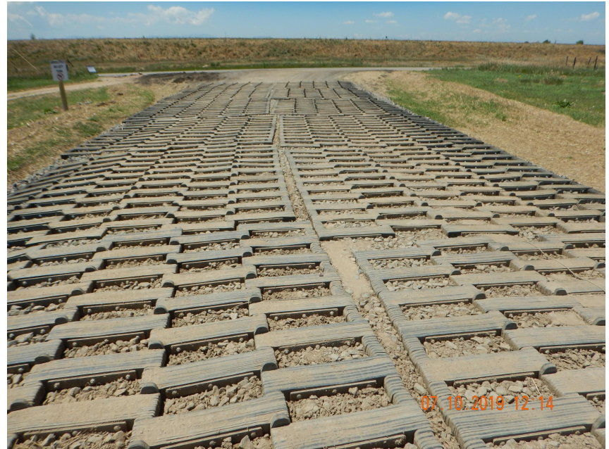
Photo 2. Photo taken from the entrance of location, facing West. Photo illustrates the second vehicle tracking device BMP.
