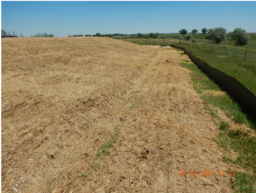
Photo 3. Photo taken from the southern location, facing East. Photo illustrates a ditch and berm BMP has been installed in conjunction with silt fence. Disturbance areas have been seeded and straw crimped with mulch.
