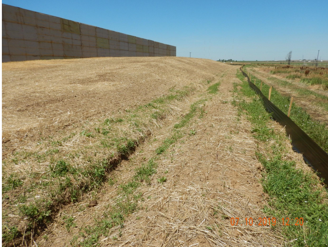
Photo 7. Photo taken from the eastern location, facing North. See comments under Photo 3. Photo also illustrates the topsoil stockpile which has been stabilized with equipment tracking, seeded, and straw crimped with mulch.
