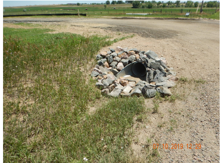
Photo 11. Photo taken from the entrance of location, facing South. Photo illustrates the culvert has been stabilized along inlet.
