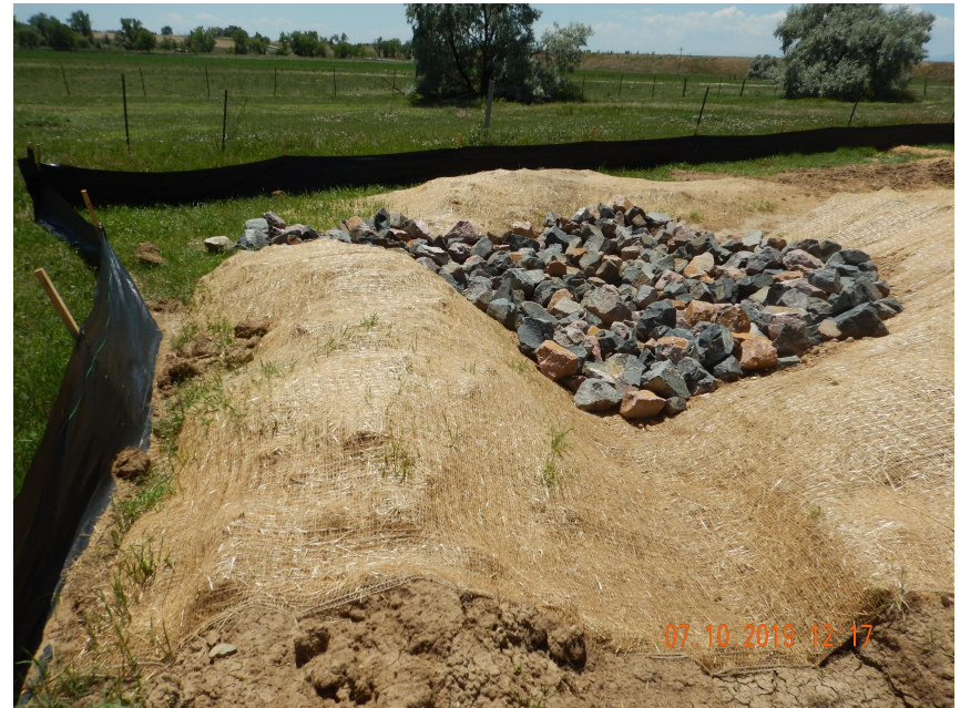
Photo 4. Photo taken from the southeastern location, facing South. Photo illustrates a sediment trap with a stabilized outlet. Embankment berms of sediment trap and adjacent areas have been temporarily stabilized with erosion control blankets.
