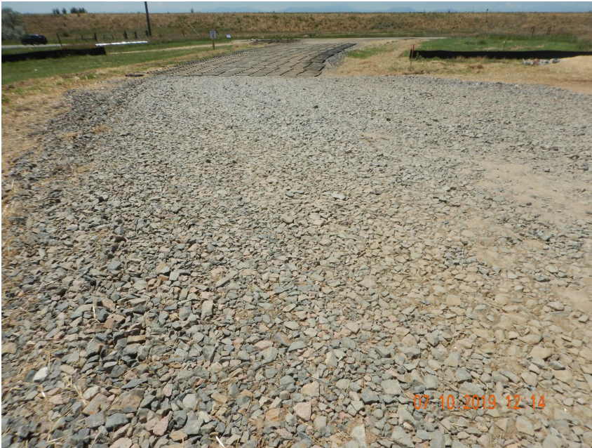
Photo 1. Photo taken from the entrance of location, facing West. Photo illustrates one of two vehicle tracking device BMPs.
