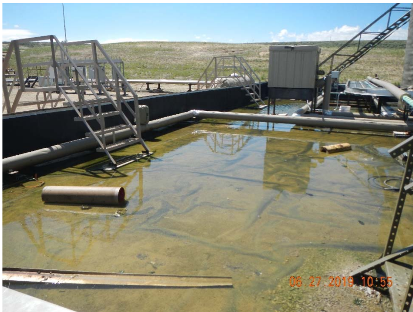
Photo 7. Trash and debris in battery berm.
