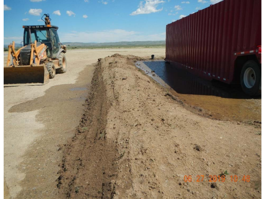
Photo 2. Water seeping through and under berm. No labels on tanks.
