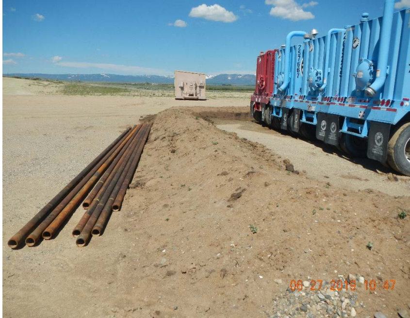
Photo 1. Tubing stored outside tank berm. No labels on tanks.
