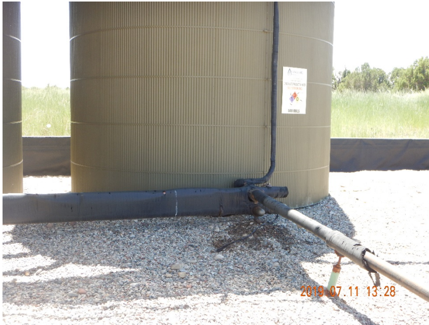
Photo #9 – Localized accumulation of oil-stained material beneath valve on southwest condensate/produced water AST.
