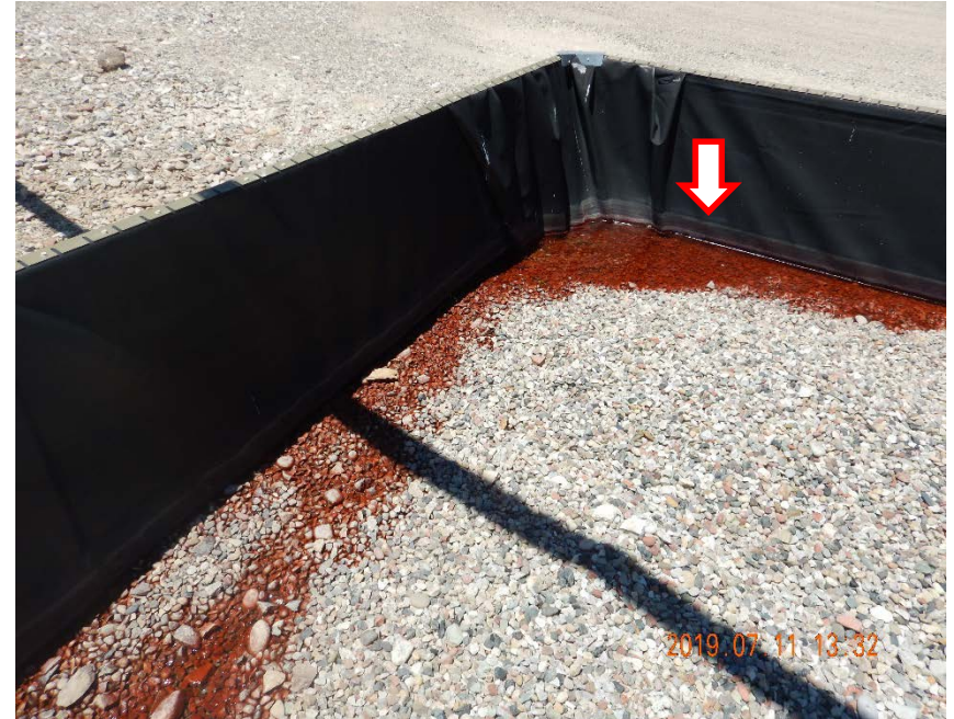
Photo #16 – Red fluid accumulation at northwest corner of tank battery secondary containment, note staining level on liner.
