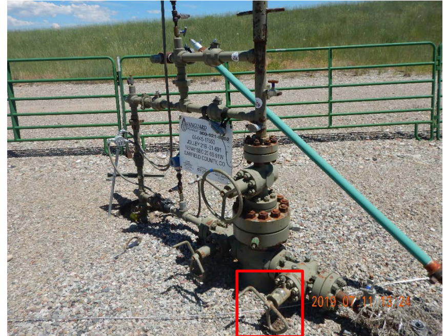
Photo #4 - Jolley 21B-21-691 wellhead. Note localized accumulation of oil-stained material beneath valve.
