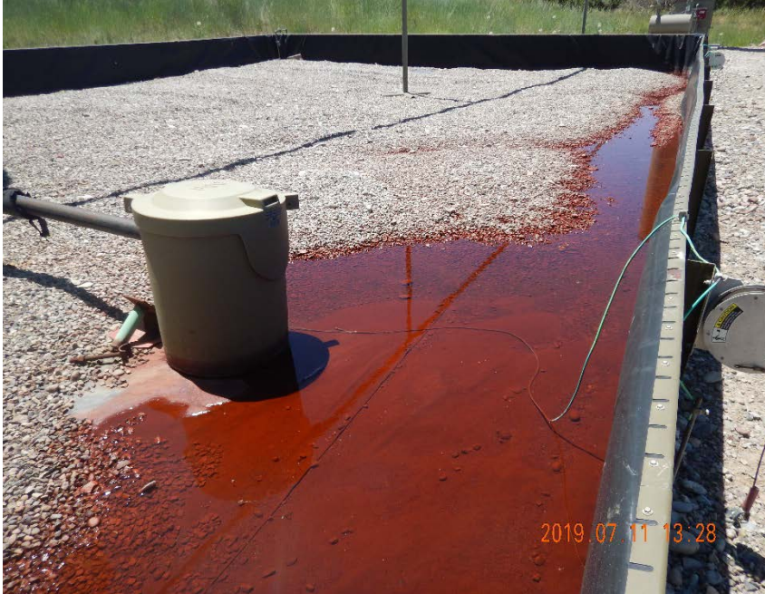
Photo #13 – Unidentified red fluid and staining inside north side of tank battery secondary containment.
