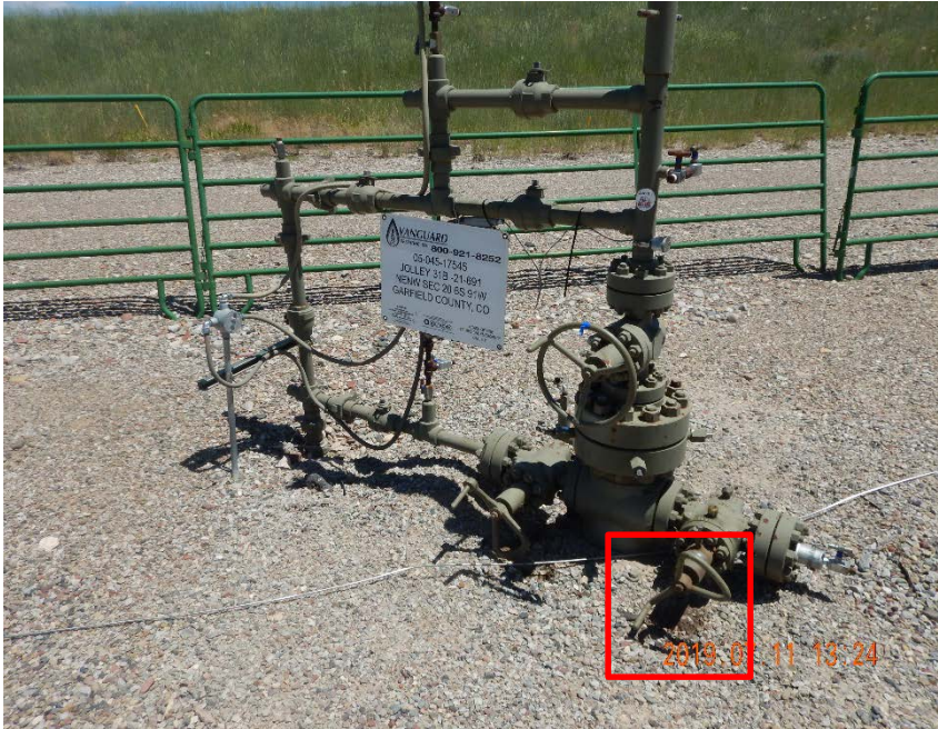
Photo #3 – Jolley 31B-21-691 wellhead. Note localized accumulation of oil-stained material beneath valve.
