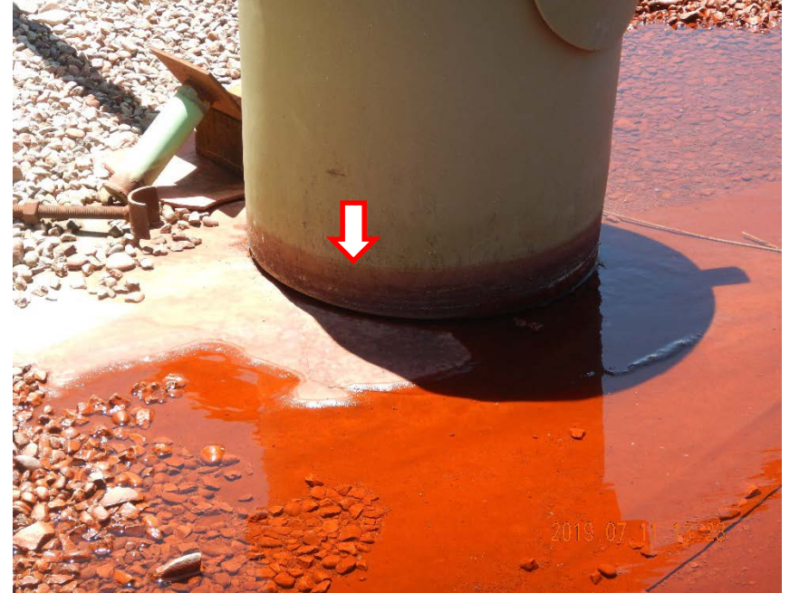
Photo #14 – Red staining on truck loadout containment device indicates previous fluid level.
