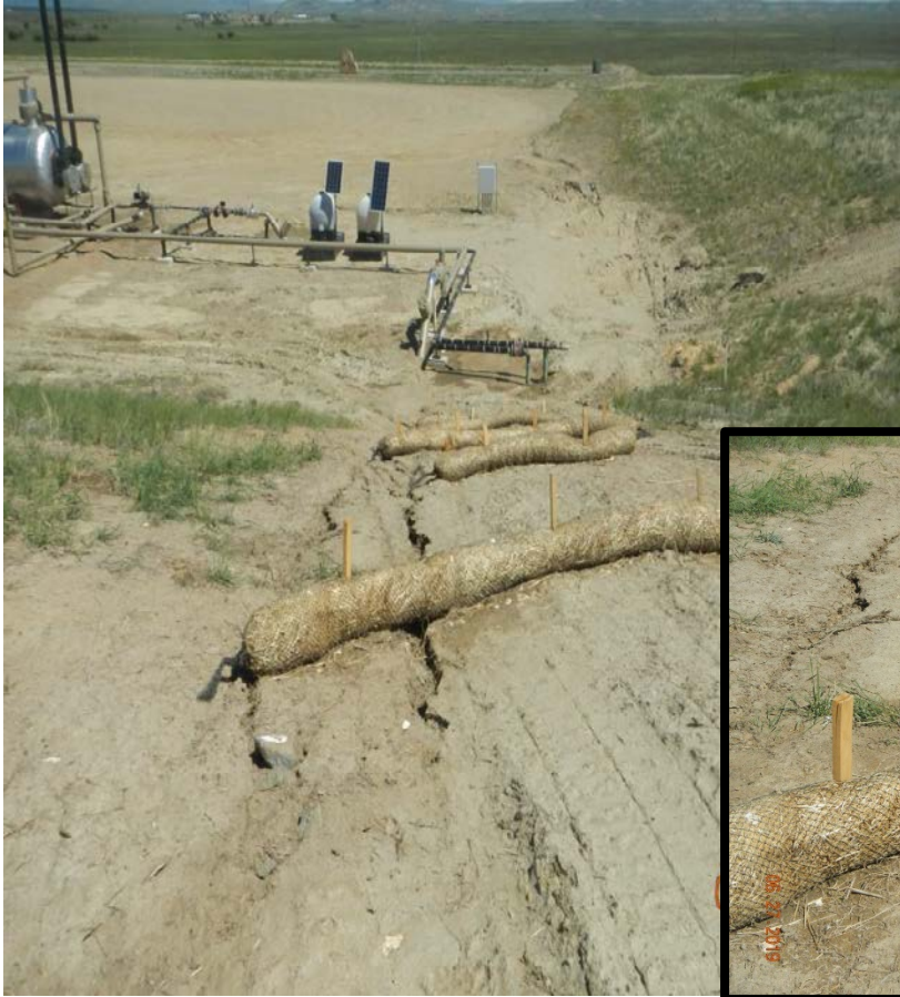
Photo#4: BMPS have failed; erosion occurring on Southeast corner of cut slope. Note undercutting of improperly seated wattles.
