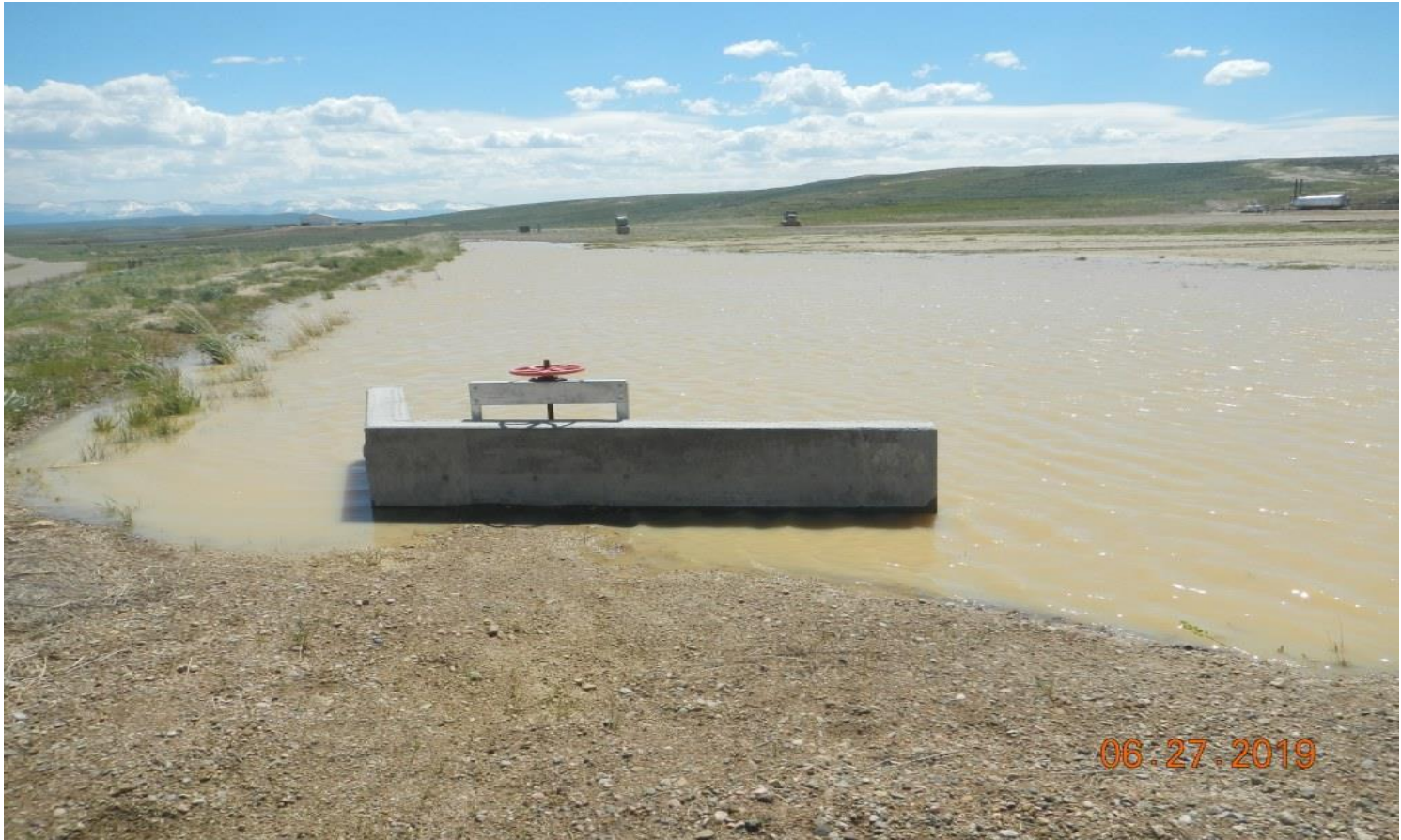
Photo#8: Weir installed at Northwest corner retaining Stormwater.
