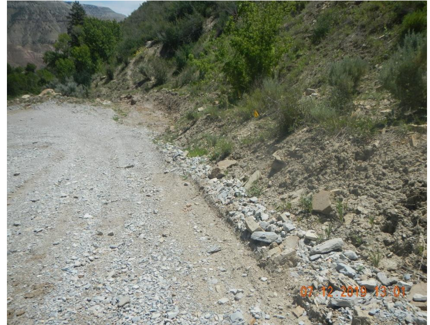
Ditch needs maintained at switch backs
