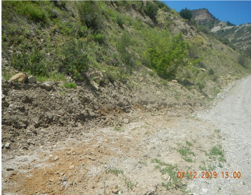
Ditch needs maintained at switch backs
