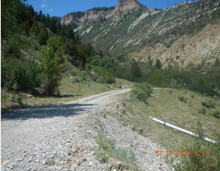
Busted PVC line plumbed into culvert(slide area)
