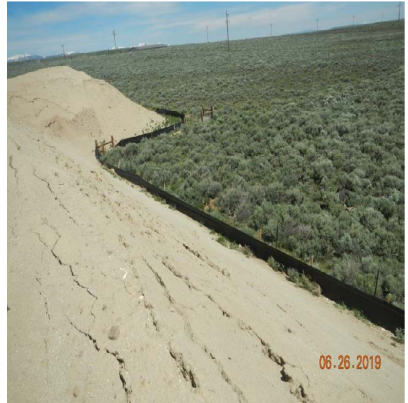
Photo#3: View along unstable stockpile pile perimeter.
