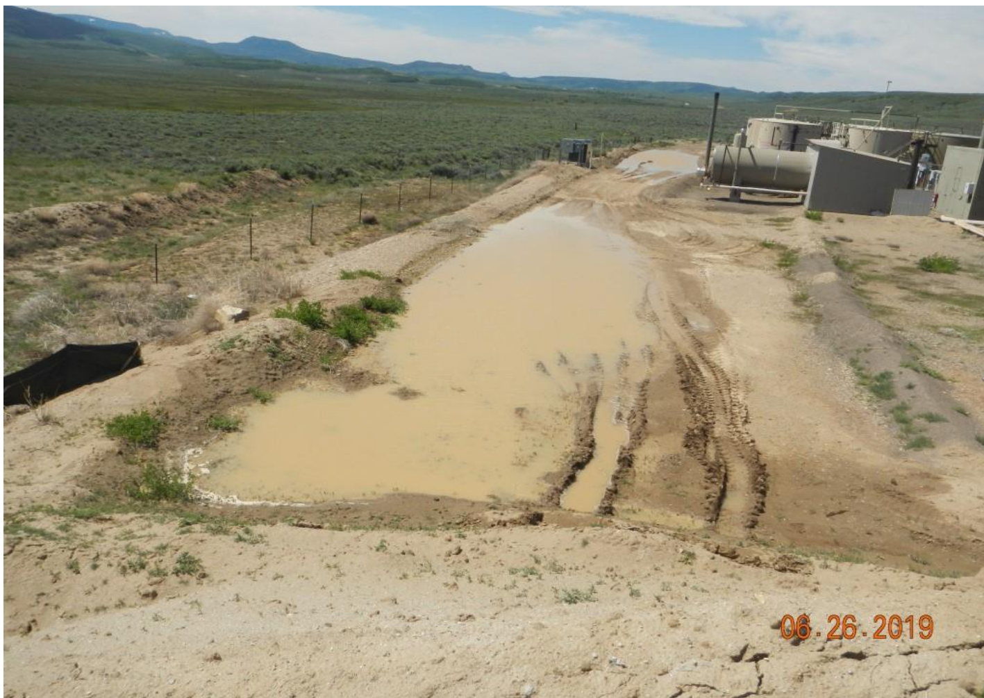
Photo#14: Stormwater is improperly ponding on East side of site.
