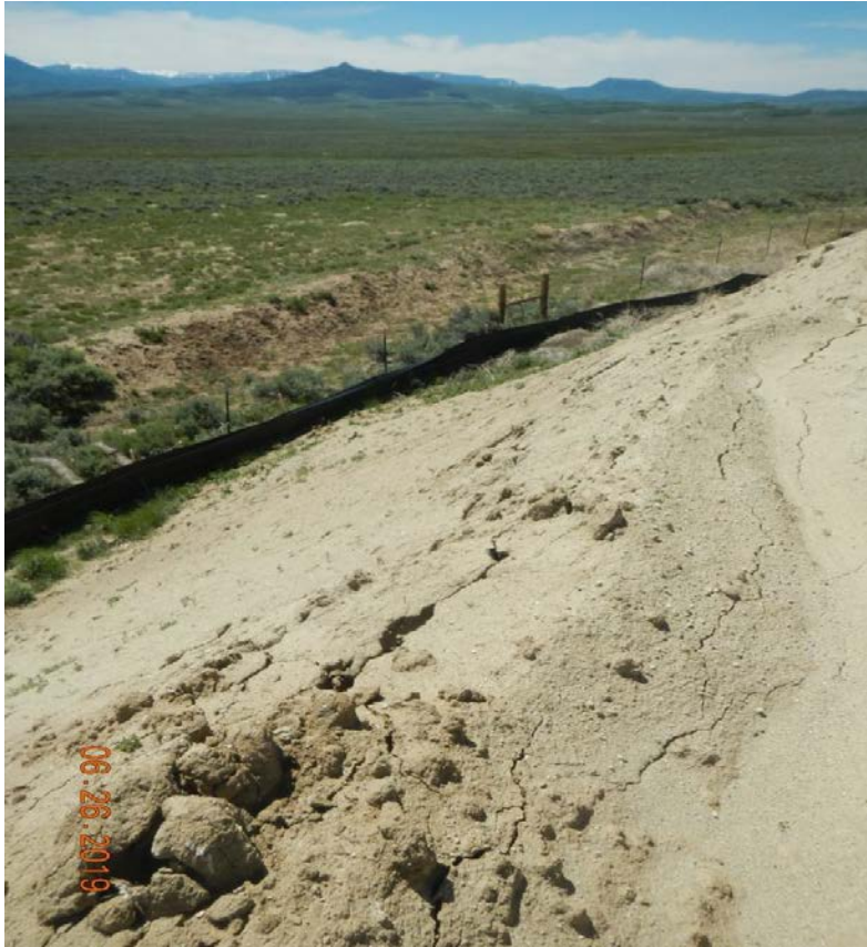
Photo#6: Cracking, sloughing, erosion of stockpile.
