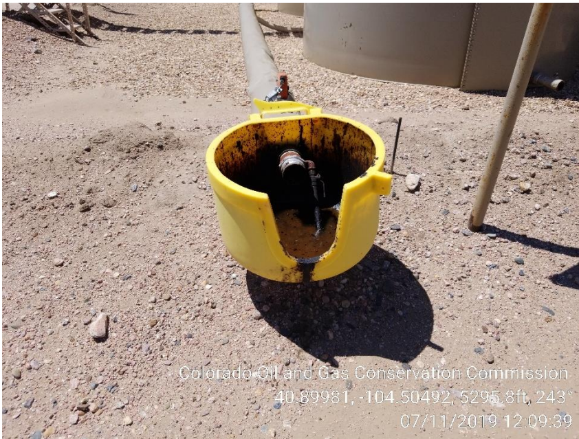
Photo 7 – South Loadline bucket missing lid
