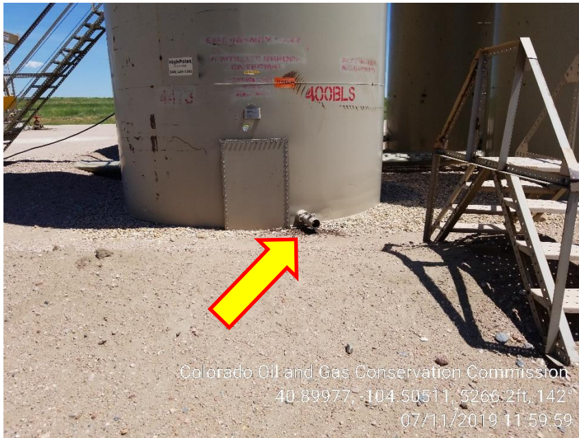
Photo 5 – Stained Soil at Northwest back bottom valve
