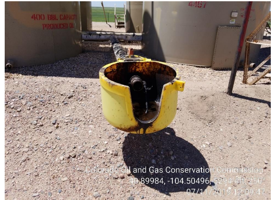
Photo 8 – North Loadline bucket missing lid
