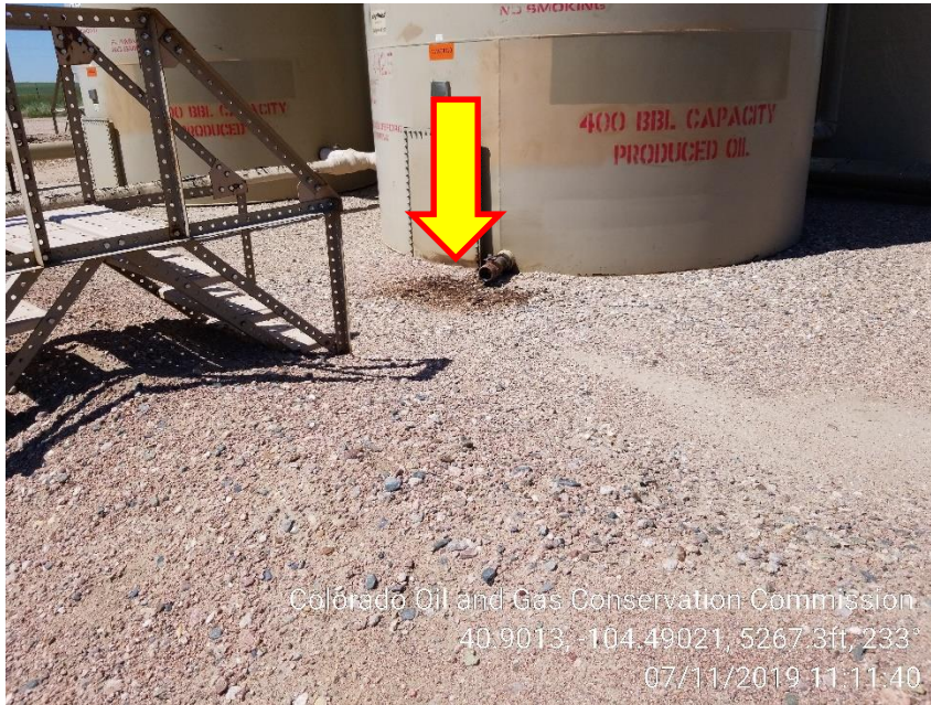
Photo 5 – Stained Soil at the Northeast Tank back bottom valve
