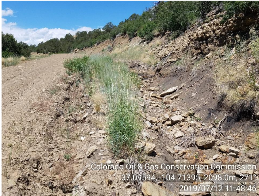
PHOTO 3: AREA OF EROSION ON MAIN ROW NORTH OF LOCATION TOWARD THE BOTTOM OF THE HILL. REPAIR EROSION AND REPAIR OR INSTALL BMP'S TO PREVENT EROSION AND COMPLY WITH RULE 1002.f. CA DATE 8/12/19
