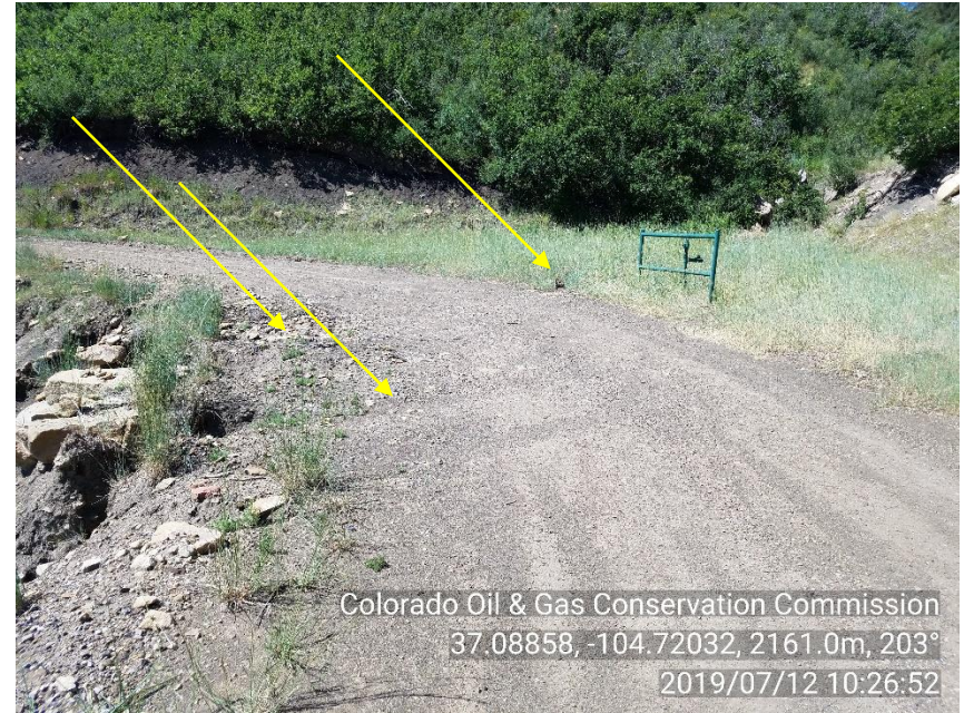
PHOTO 6: ANOTHER AREA APP. 200 YARDS SOUTH FROM PREVIOUS PHOTOS OF NO DITCHING OR BERMING ON ROW TO PREVENT STORMWATER CAUSING ROW SURFACE MATERIAL TO MIGRATING OFF OF ROW AND BEYOND ORIGINAL ROW DISTURBANCE AREA. INSTALL OR REPAIR BMP'S TO PREVENT STORMWATER POOLING ON ROW AND TO PREVENT ROW SURFACE MATERIAL FROM MIGRATING OFF OF ROW IN ACCORDANCE WITH RULE 1002.f. CA DATE 9/12/19.
