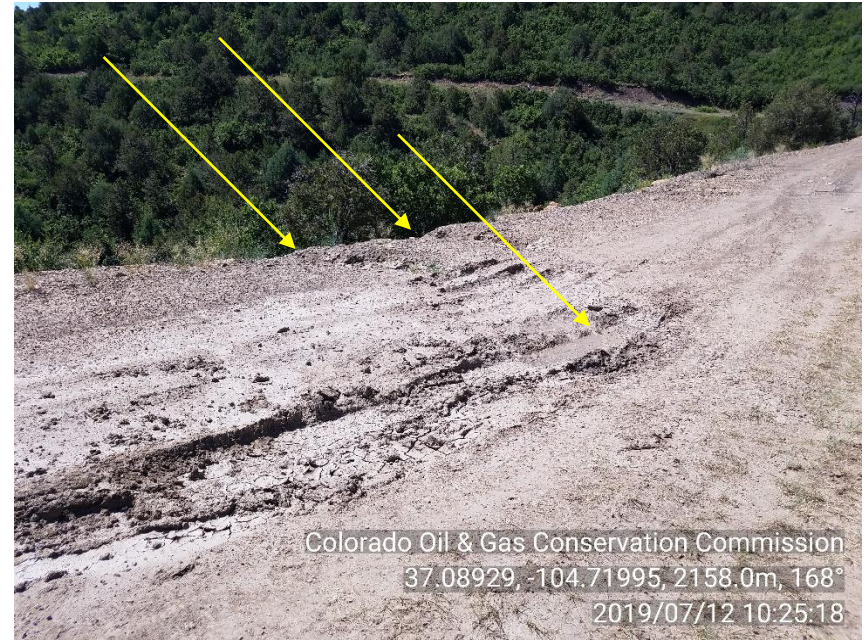
PHOTO 4: CLOSER VIEW FROM PREVIOUS PHOTO (PHOTO 3). PHOTO SHOWING STORMWATER POOLING ON ROW AND EROSION OF ROW SURFACE MATERIAL OFF OF ROW.
