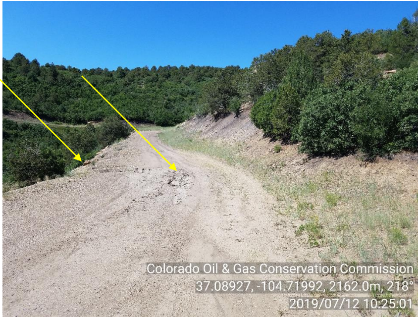
PHOTO 3: NO DITCHING OR BERMING ON ROW TO PREVENT STORMWATER POOLING ON ROW AND ROW SURFACE MATERIAL FROM MIGRATING OFF OF ROW AND BEYOND ORIGINAL ROW DISTURBANCE AREA. INSTALL OR REPAIR BMP'S TO PREVENT STORMWATER POOLING ON ROW AND TO PREVENT ROW SURFACE MATERIAL FROM MIGRATING OFF OF ROW IN ACCORDANCE WITH RULE 1002.f. CA DATE 9/12/19.
