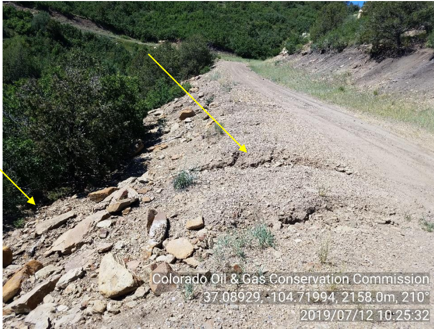
PHOTO 5: CLOSER VIEW OF ROW EROSION AND ROW SURFACE MATERIAL MIGRATION OF ORIGINAL ROW DISTURBANCE AREA FROM THE PREVIOUS 2 PHOTOS (PHOTO'S 3 & 4).
