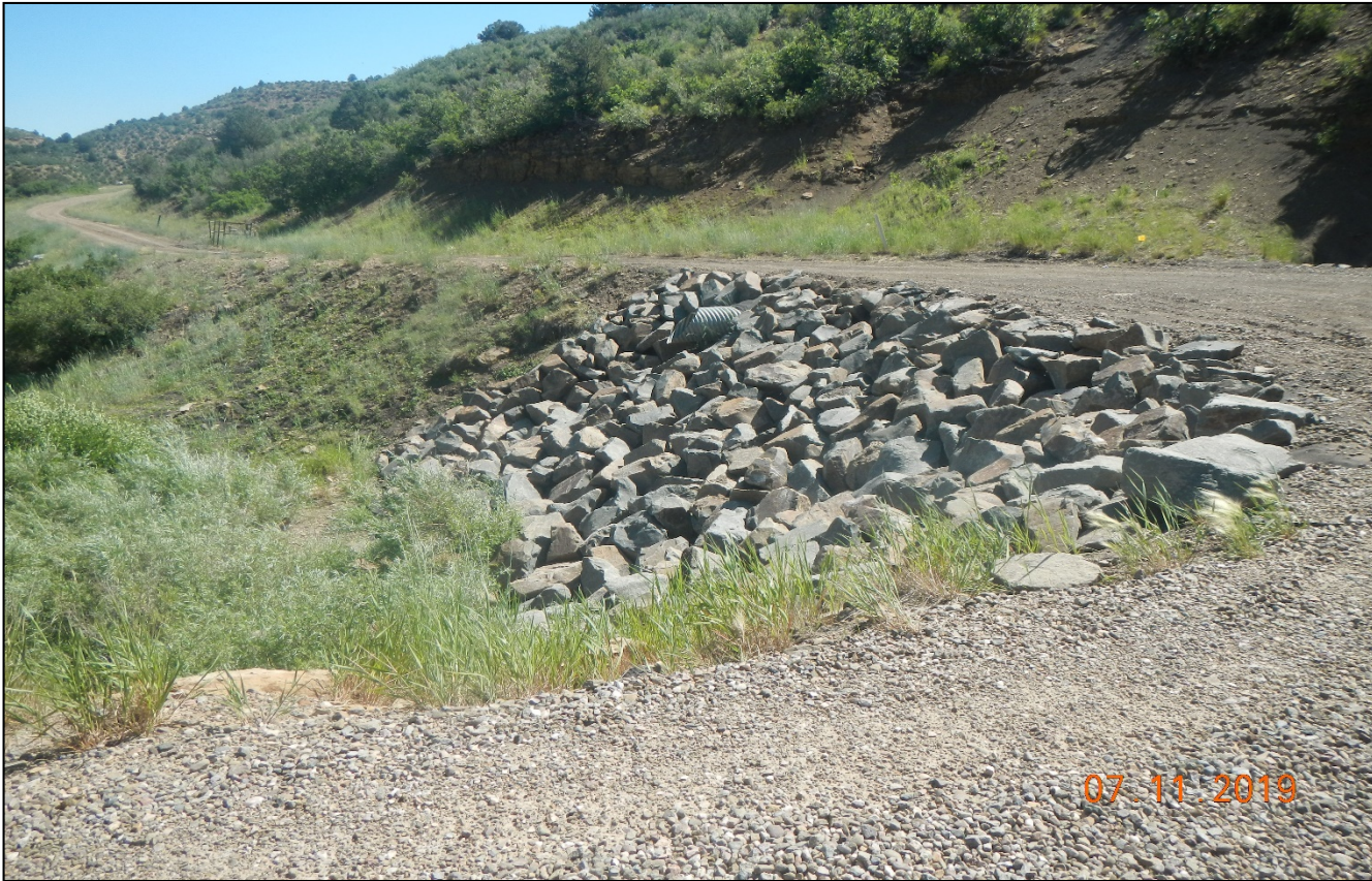
Photo 2. Facing along the access road. Rock rip/rap has been installed in areas of erosion.
