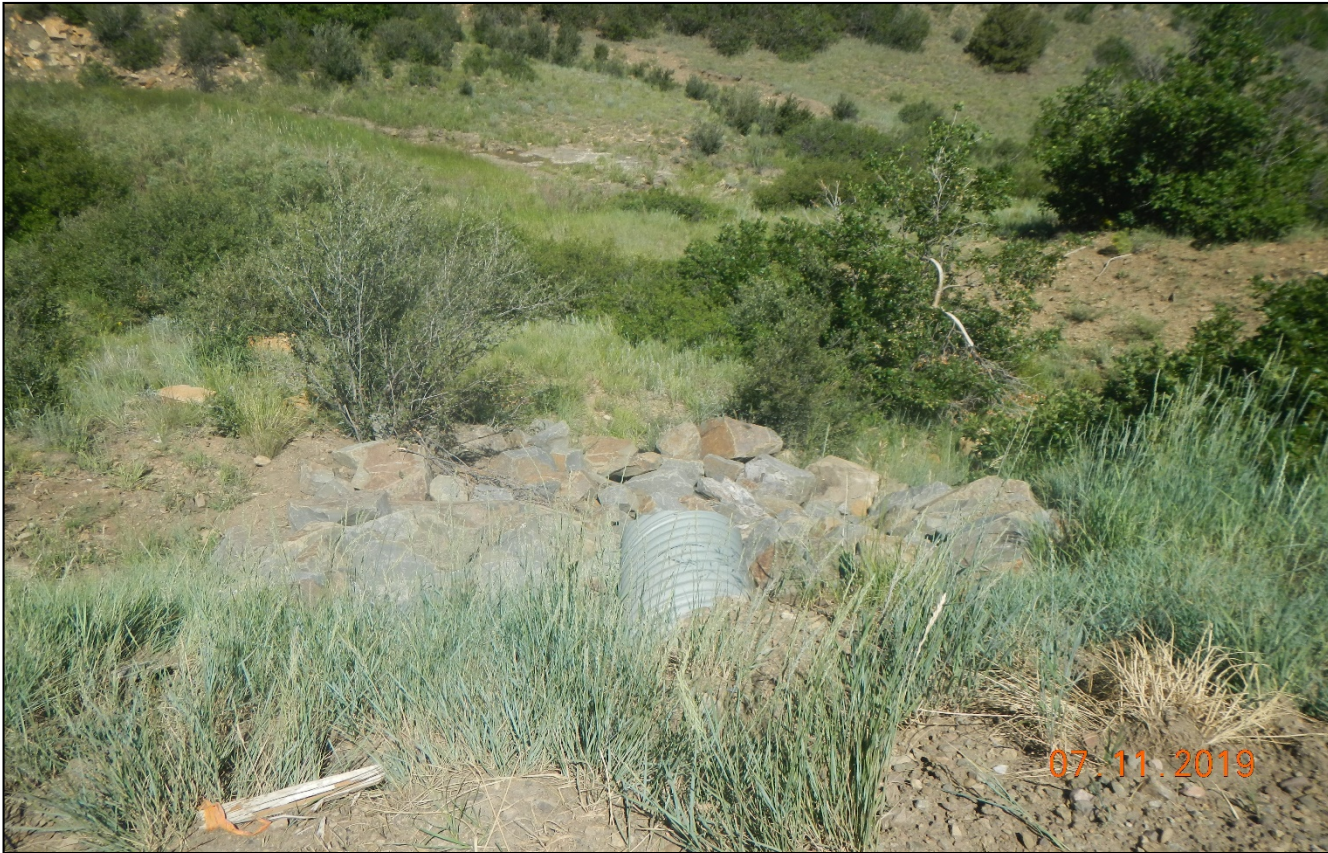
Photo 3. Outlet protection has been installed on the culvert.
