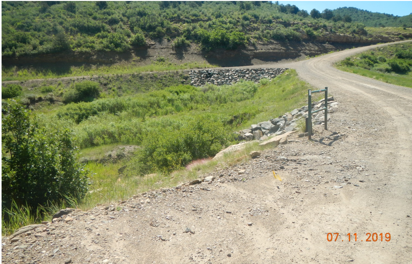
Photo 1. Facing along the main road. Rock rip/rap has been installed in areas of erosion.
