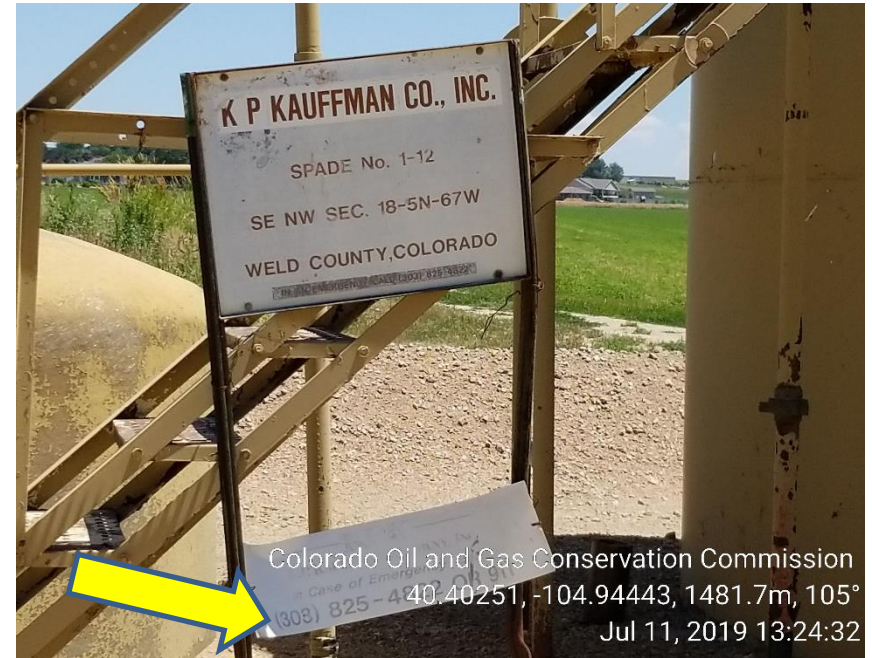
Photo 2: Battery sign; significant fading of emergency contact number.
