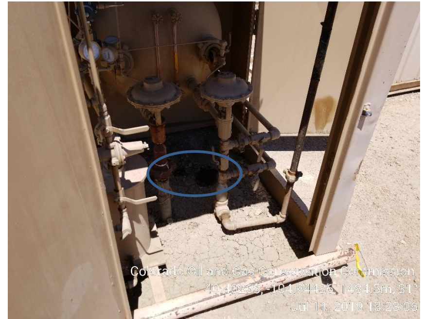
Photo 8: Stained soil in separator house.
