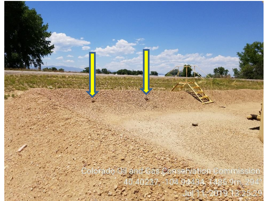
Photo 6: Holes inside berm wall
