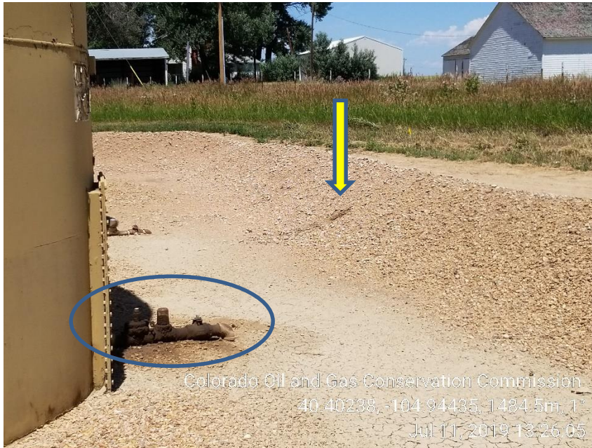
Photo 7: Stained soil; hole inside of berm
