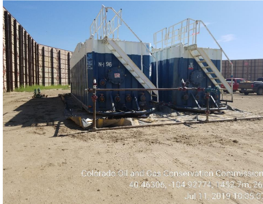
Photo 1: No grounding rod present
