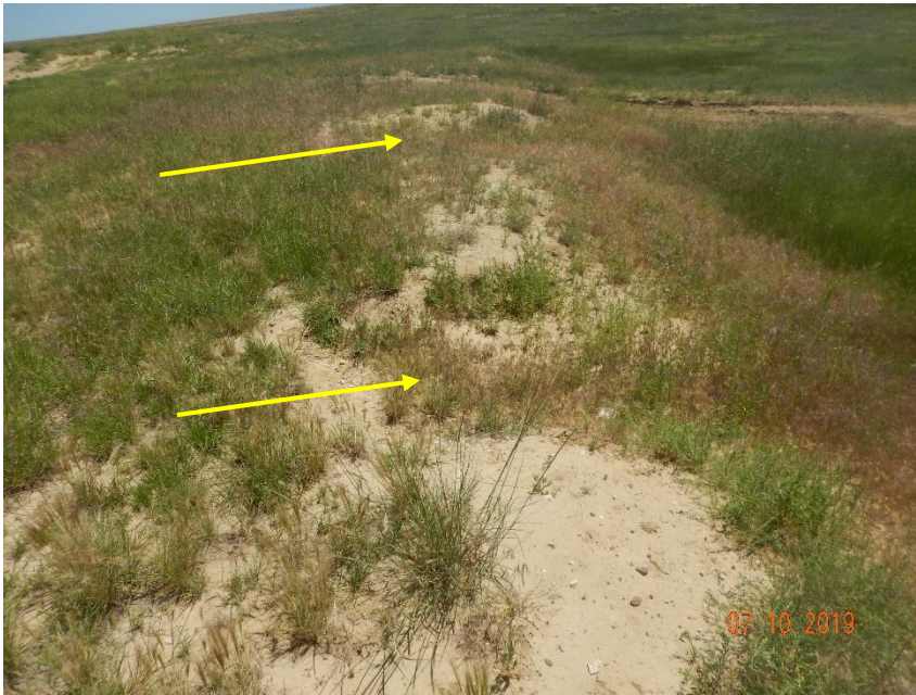
Photo 17: Photo taken from the south end of the location, facing east. Previous inspections documented erosion degradation on the location and required operator to implement BMPs in accordance with 1002.f. Photo shows erosion degradation remains, no BMPs have been installed or maintained.
