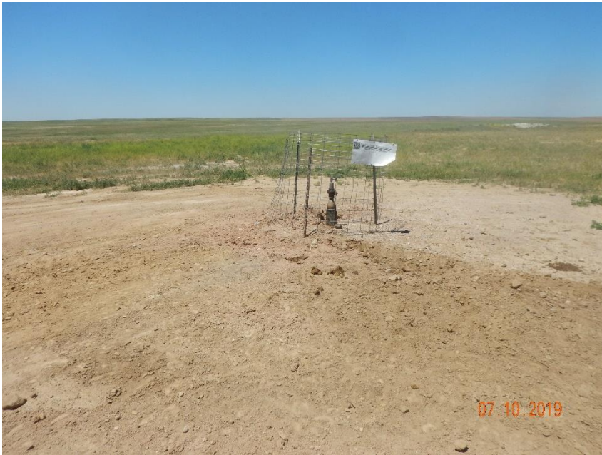
Photo 1: Photo taken from the well. Photo shows pump unit has been removed.
