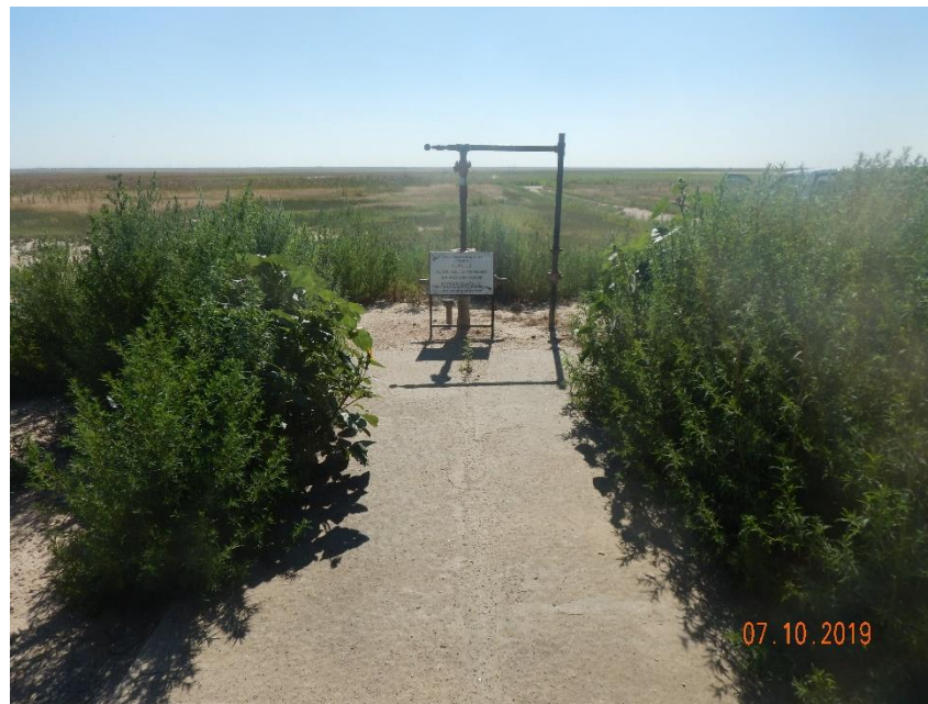
Photo 4: Photo shows weed accumulation around production equipment.
