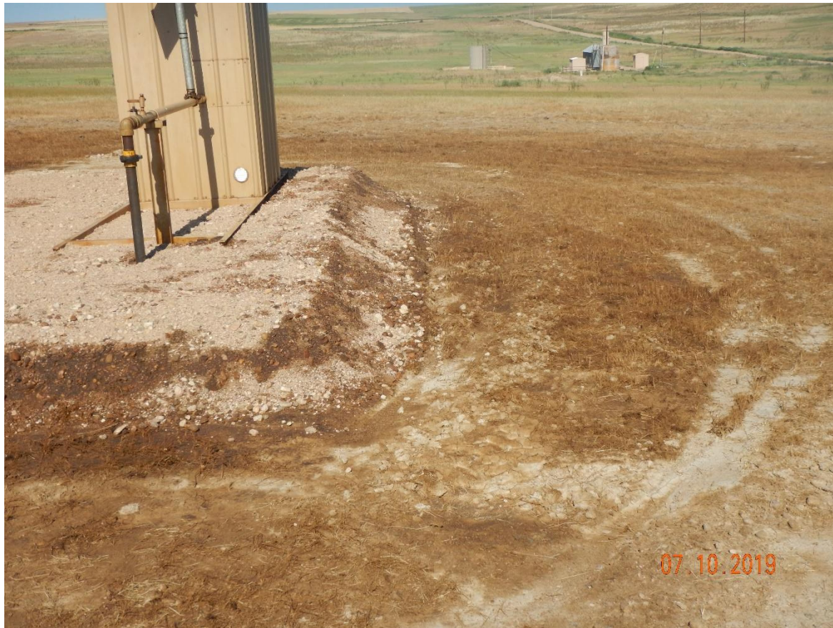
Photo 5: Photo taken from the meter runs on the west end of the location, facing west. Photo shows stained soils at the meters and adjacent lands
