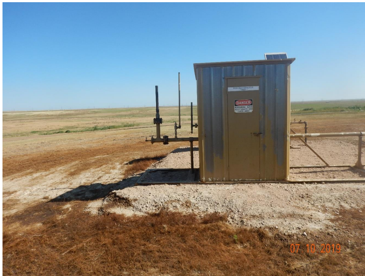
Photo 1: Photo of meter runs on the west end of the location. Gas freely venting from the meter.
