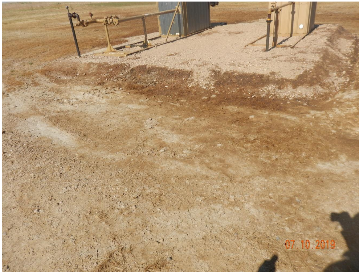
Photo 3: Photo taken from the meter runs on the west end of the location, facing west. Photo shows stained soils at the meters and adjacent lands
