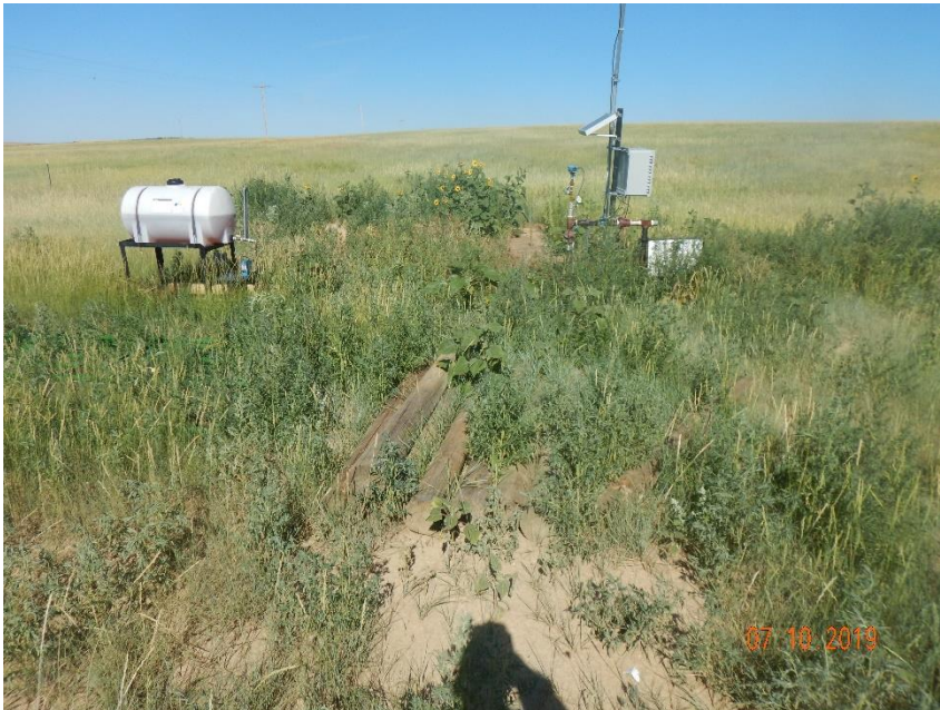
Photo 1: Photo taken from the location, facing west. Photo shows weedy vegetative growth has established/accumulated around the well and production equipment; This is considered a fire hazard and needs to be removed.
