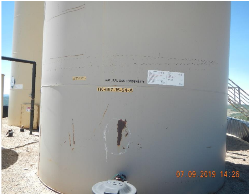
Photo 9 Tank has contents post as both Condensate and Produced Water.
