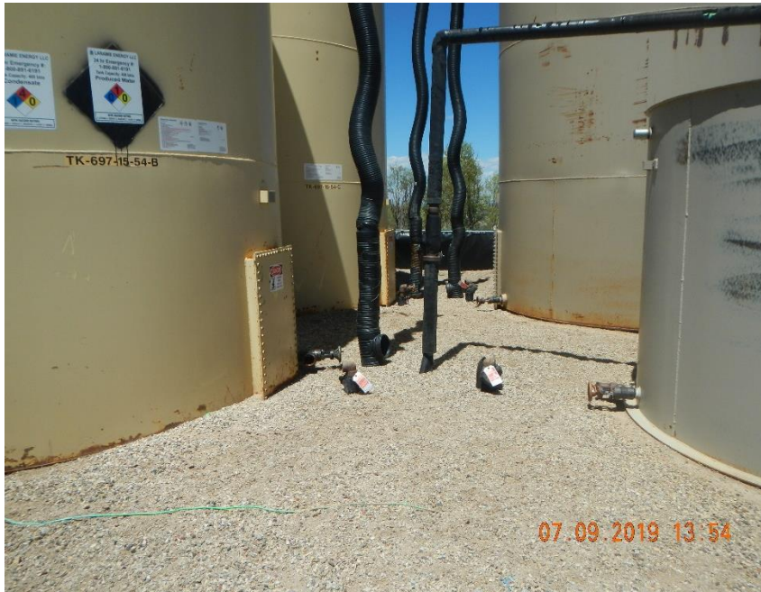
4-2" risers in tank battery with lock out tags have no plugs.
