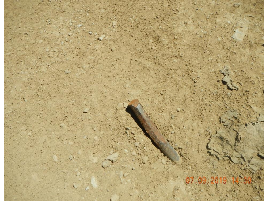
Photo 6 Unmarked guy line anchor.
