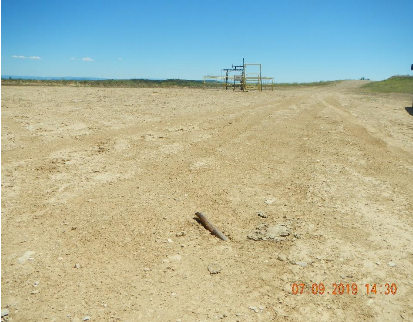
Photo 5 Unmarked guy line anchor.
