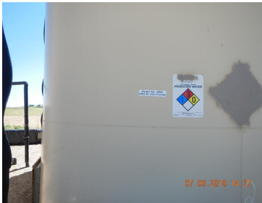
Photo 13 Producing water label with NFPA Fire Hazard of 3
