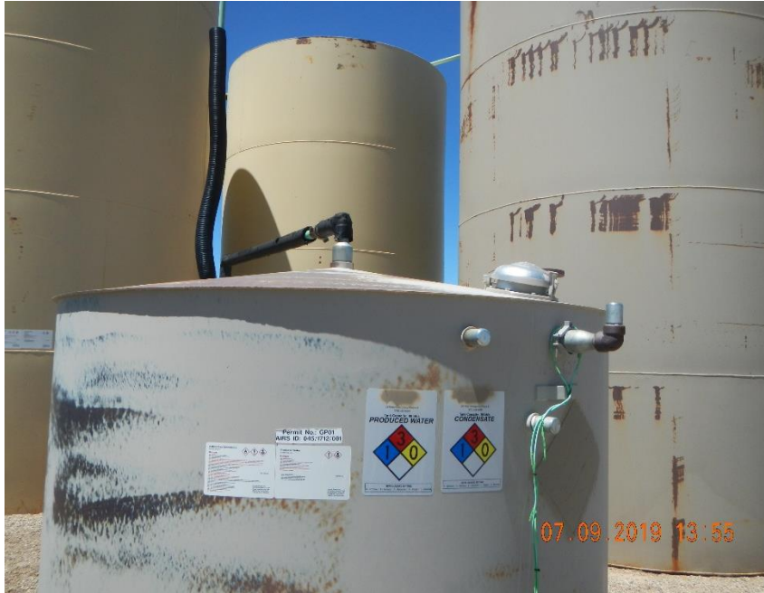
Photo 7 Open port on top of tank.
