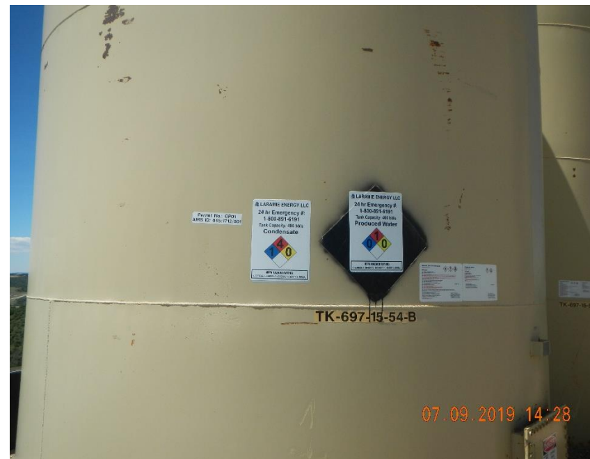
Photo 14 Condensate label with NFPA Fire Hazard of 4 next to a Producing water label with NFPA Fire Hazard of 1 on same tank.
