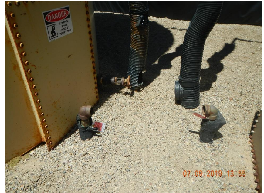
4-2" risers in tank battery with lock out tags have no plugs.
