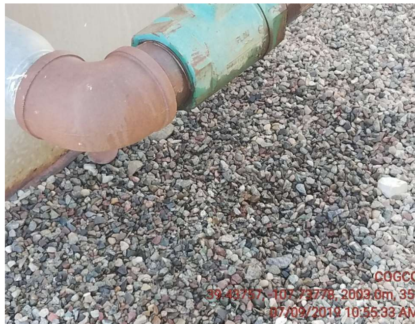
4 At time of inspection I observed a leak from the load out line on tank #1 inside the tank battery
