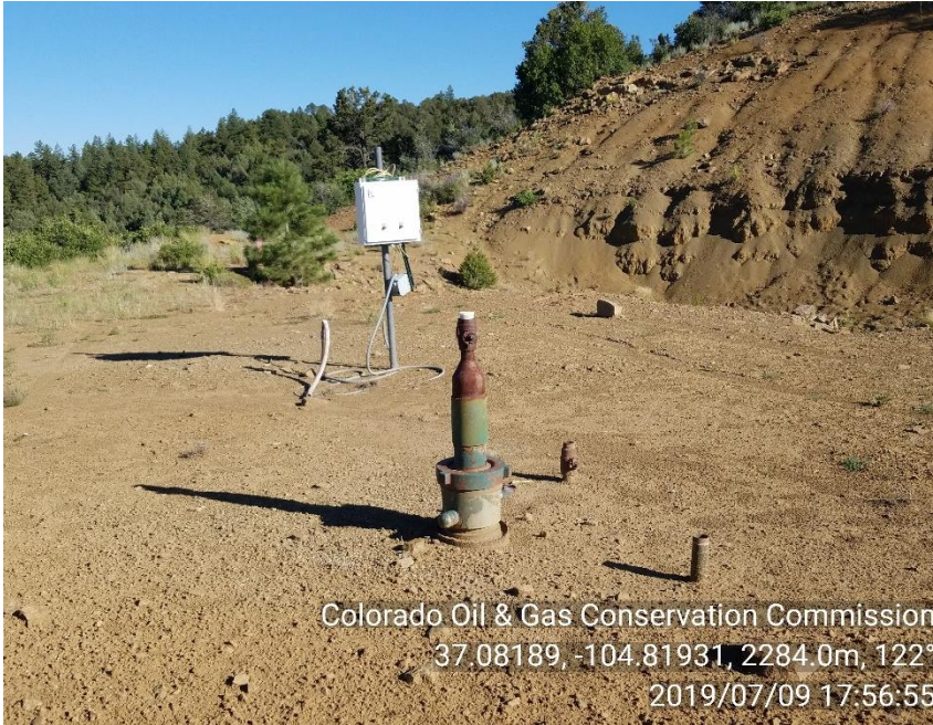
PHOTO 1: WELLHEAD/ UNUSED EQUIPMENT (TWO 2" RISERS, ONE 1" RISER AND TELEMTRY EQUIPMENT ON LOCATION). REMOVE UNUSED EQUIPMENT IN ACCORDANCE WITH NTO AND WITH RULE 603.f. CA DATE 10/9/19
