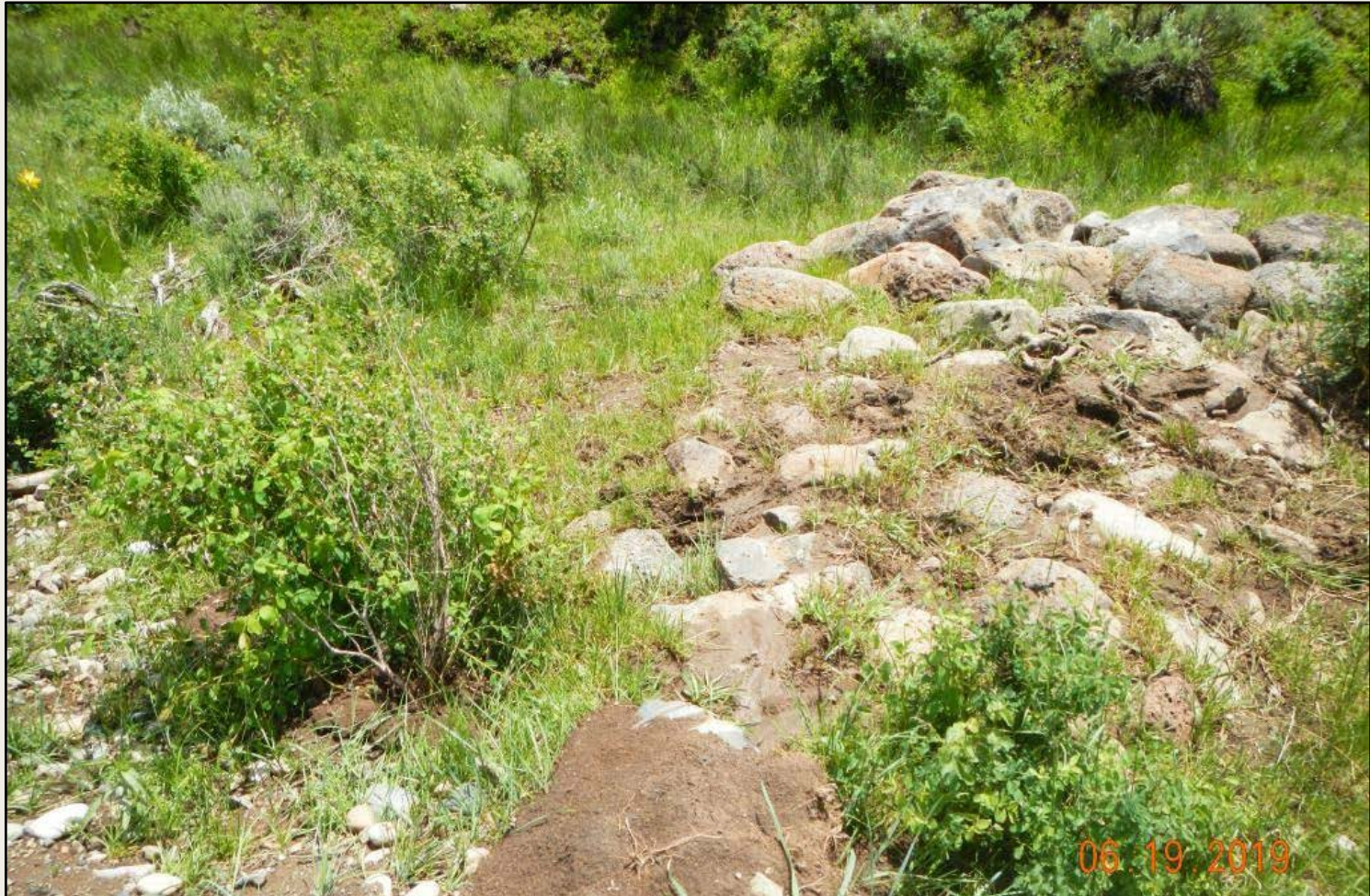
Photo 5. View of armoured culvert outlet along the access road facing downslope. Sediment in the foreground and on rocks is deposited from the culvert outlet. A perennial stream flows down-slope in the background.
