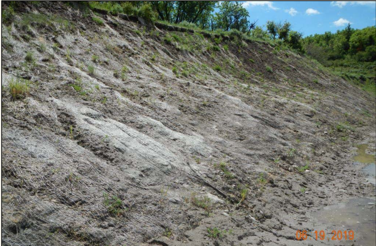
Photo 1. View of the eastern project area from the northeastern corner facing southward. Blanketing is torn and erosion is continuing.
