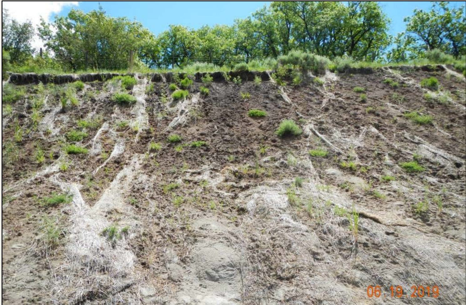
Photo 2. Another view of the eastern cut-slope with exposed soils and torn erosion control blanket.
