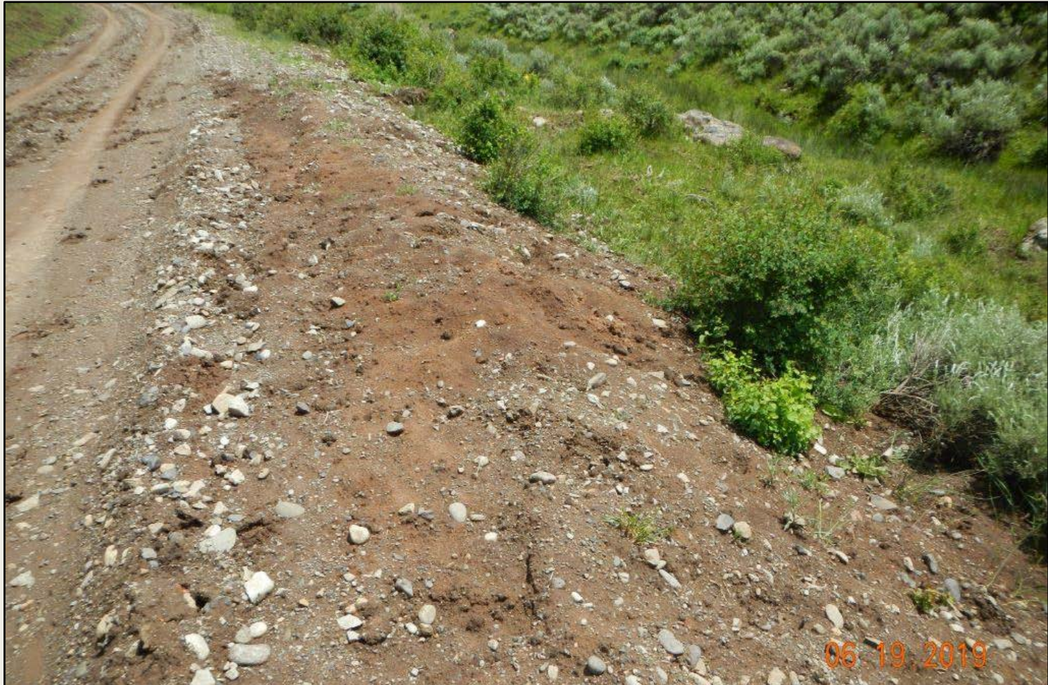
Photo 8. Another view of loose soils along the access road where soils are actively eroding downslope into the adjacent perennial stream.
