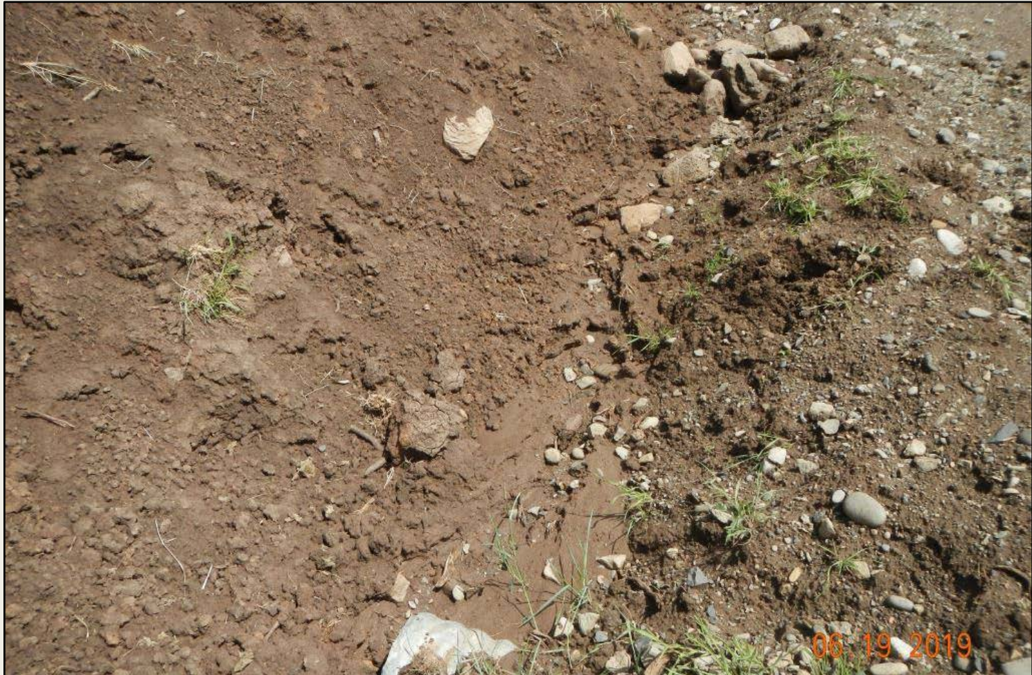
Photo 4. View of culvert and bare soils along the access road. Culvert is full of sediment and bare soils are not stabilized. Erosion is occurring within the roadside ditch.
