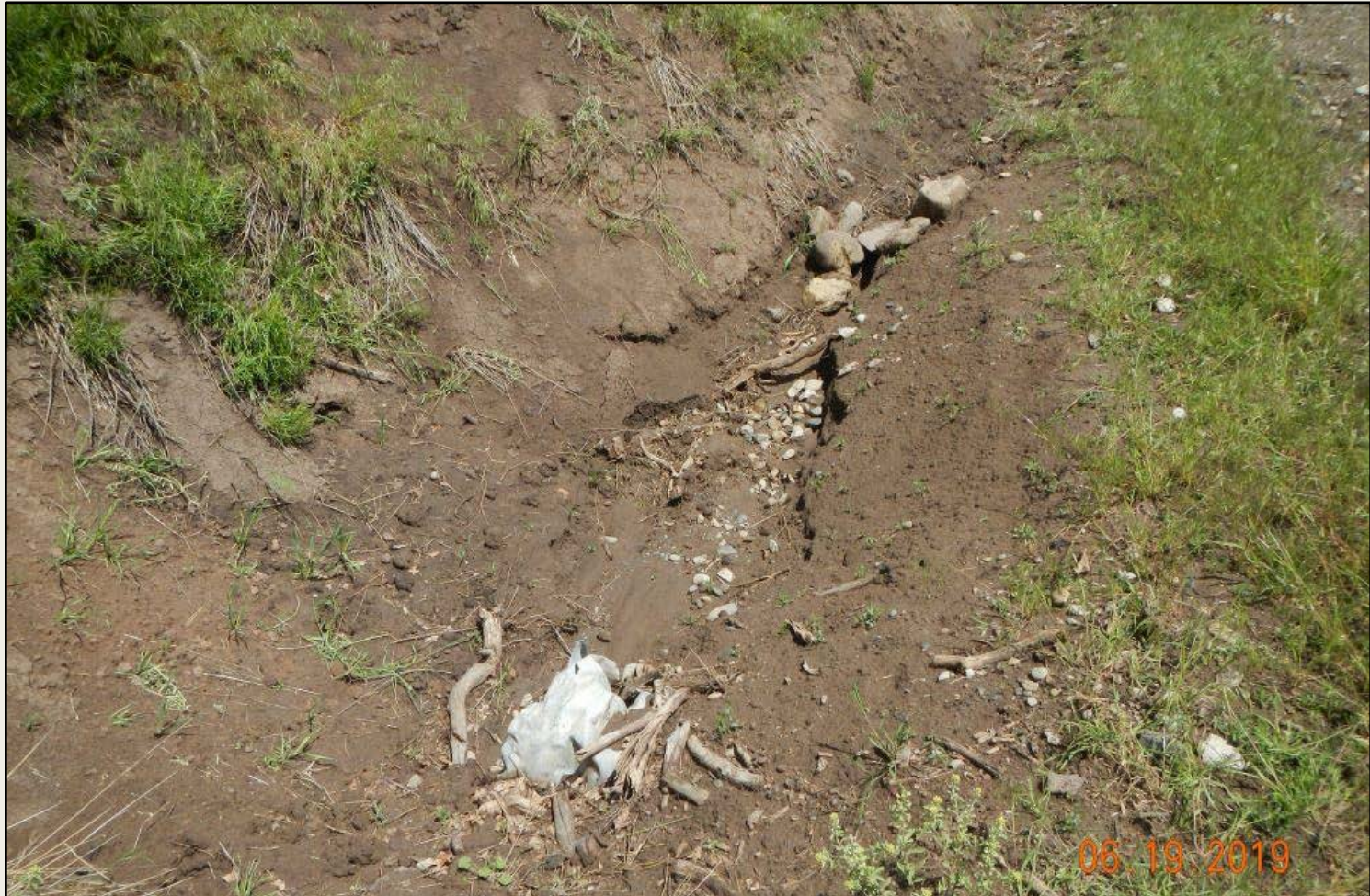
Photo 7. View of another culvert inlet along the access road. Culvert is full, drainage and loose soils on side slopes are not stabilized.
