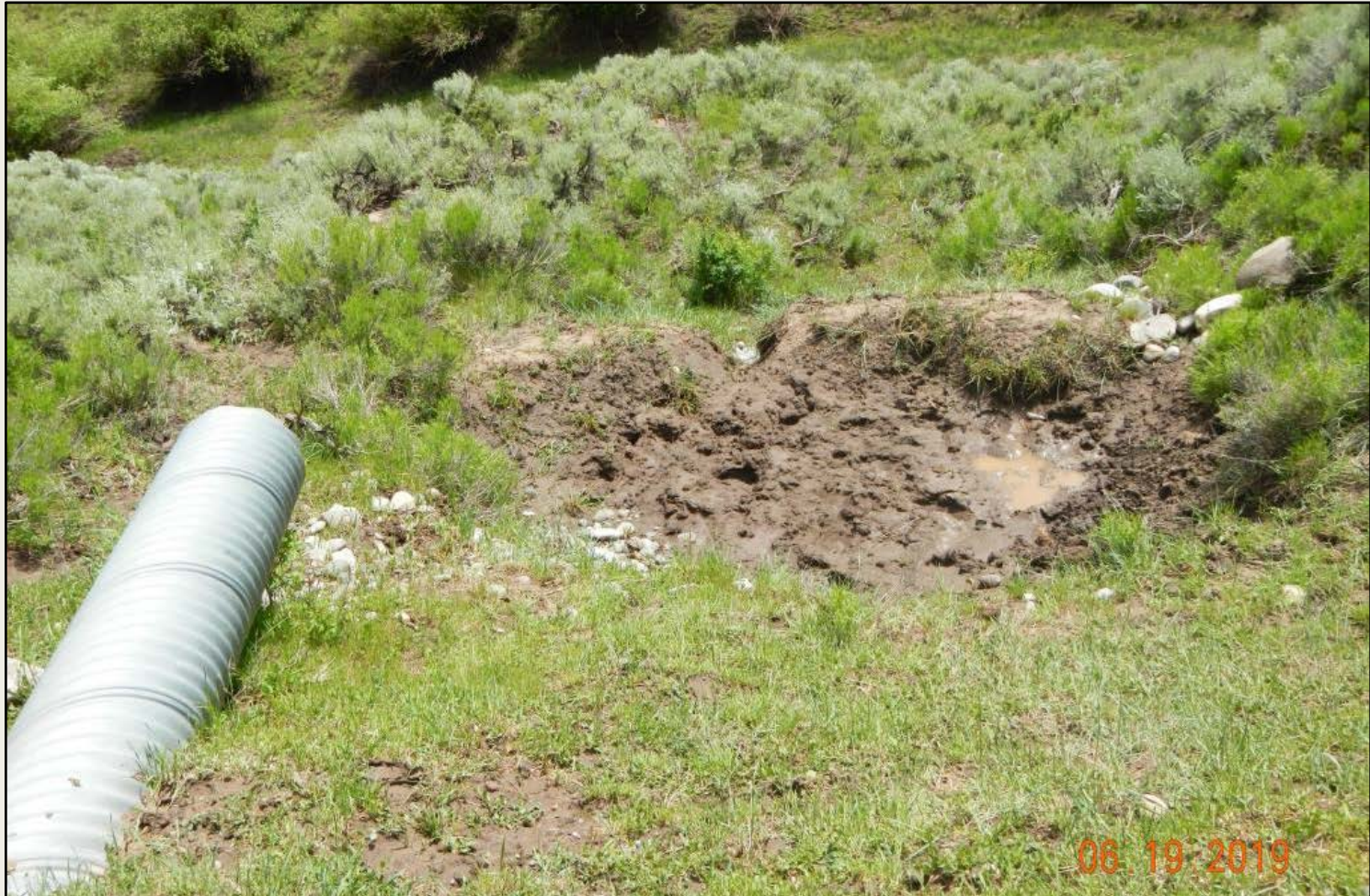
Photo 5. View of silt trap that is full of sediment and not stabilized. Culvert is installed above grade.
