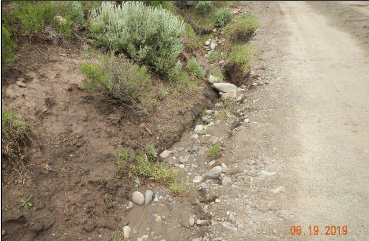
Photo 4. View of erosional channeling along the access road.
