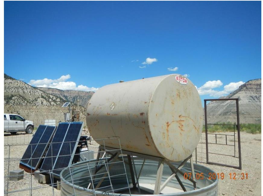
**Tank is missing Operator Name, Number, and Tank Volume.**
