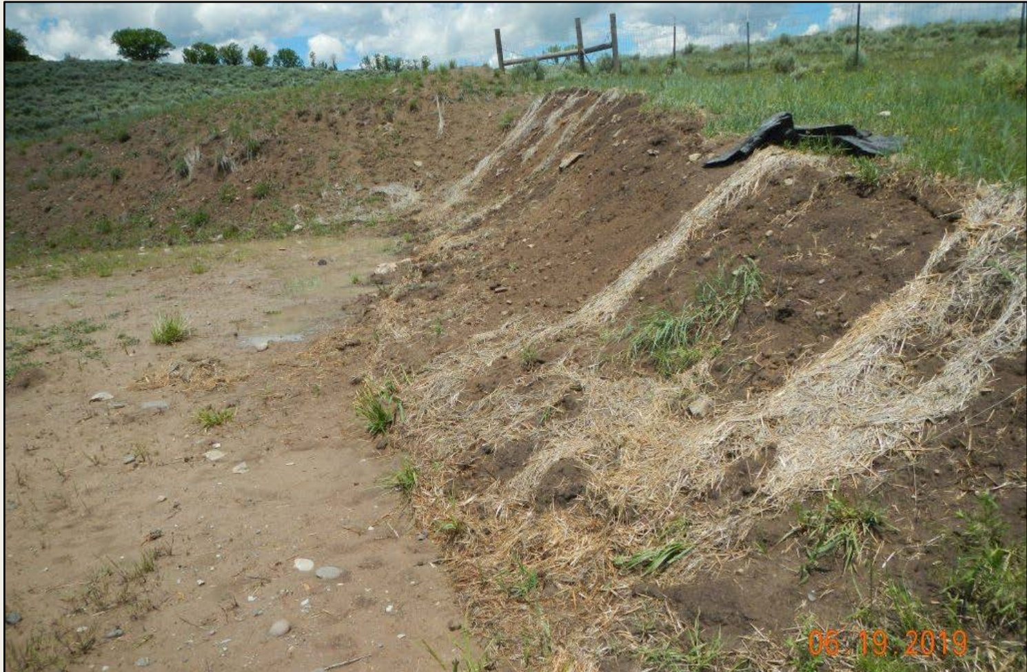
Photo 1. View of the northeastern cut-slope from the well pad entrance facing northward. Erosional blankets are torn and need repair or replacement.
