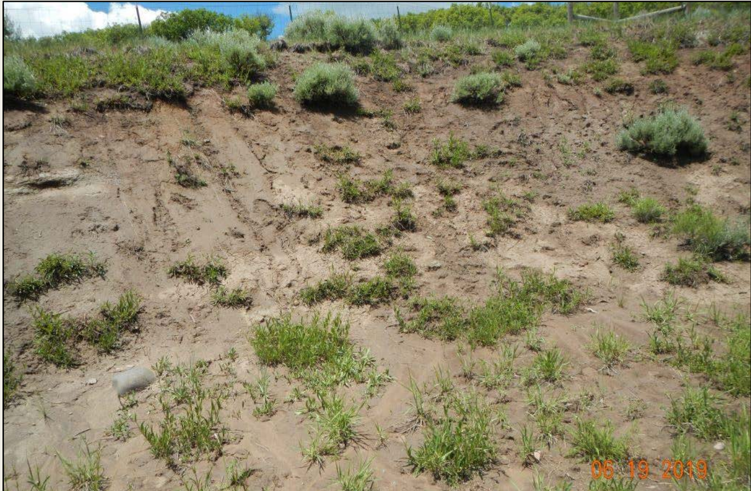
Photo 2. View of rilling within the northern cut-slope.
