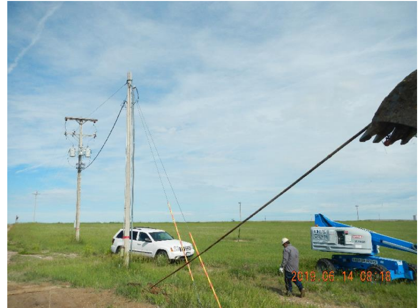
Photo 4: Pulling conduit and line.
