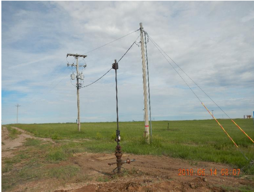
Photo 1: Wellhead with power pole to be abandoned in background. Pole will be removed by utility company.
