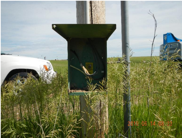
Photo 5: Line cut at the power pole drop box.
