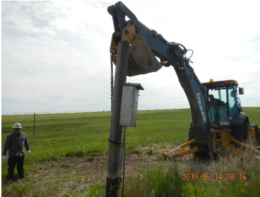
Photo 3: Pulling power control box, conduit and line.
