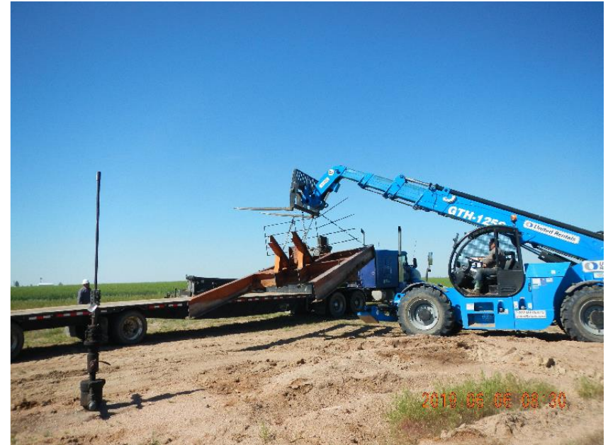
Photo 2: Loading section of pumping unit base.
