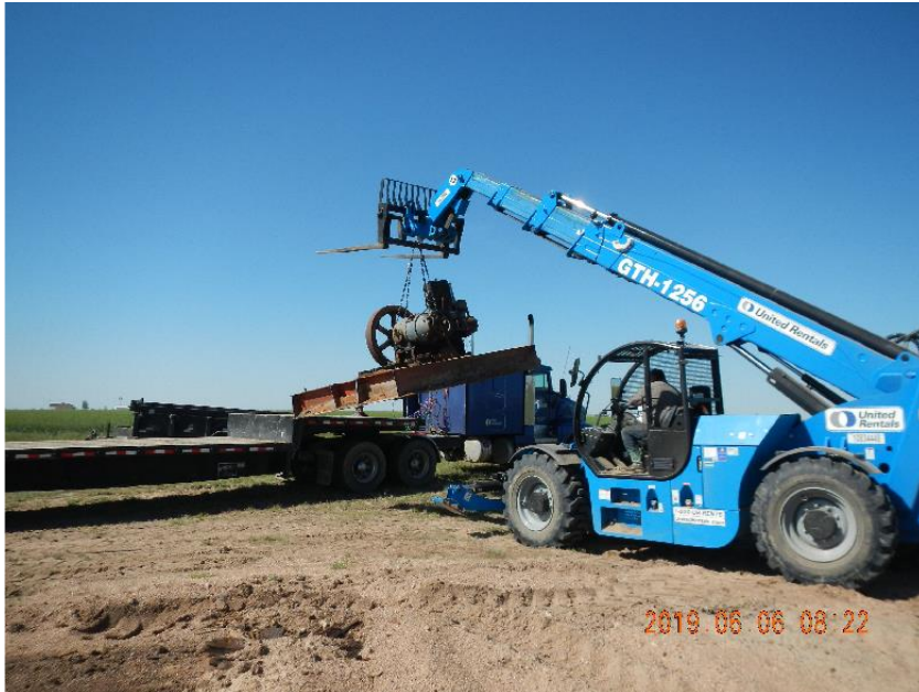
Photo 1: Loading prime mover on flatbed trailer for haul off.
