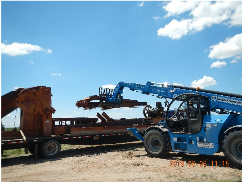
Photo 5: Loading pitman arm section.
