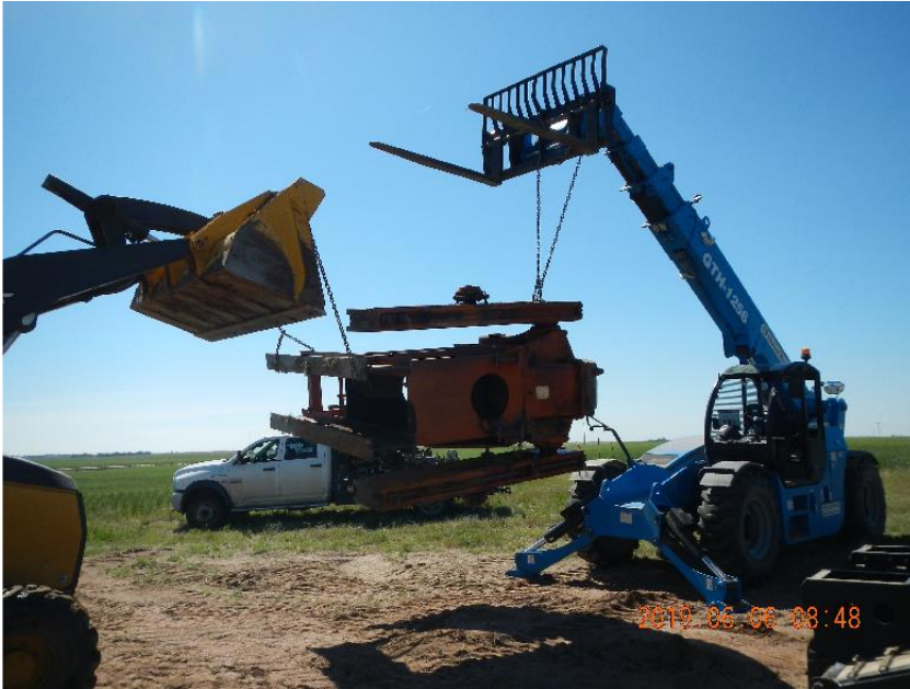
Photo 3: Lifting gear box for loading.
