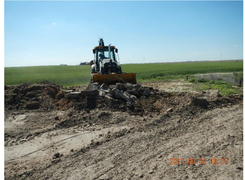
Photo 8: Backhoe scooping up concrete debris for loading.
