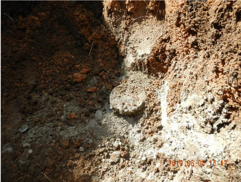
Photo 7: Cement plugged wellhead flow line.
