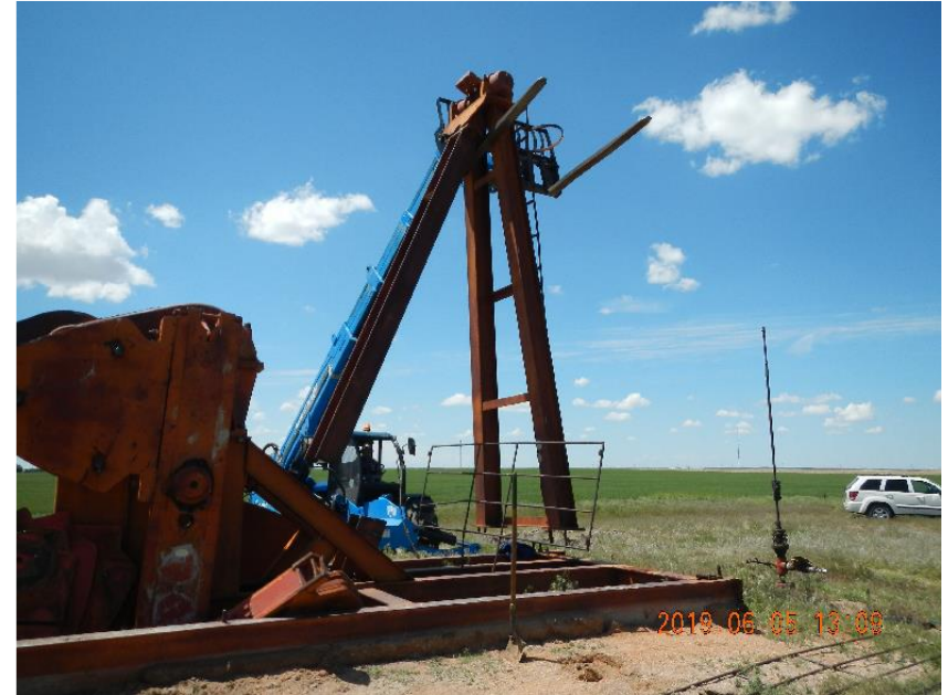
Photo 2: Removing cut off A-Frame from pumping unit base.
