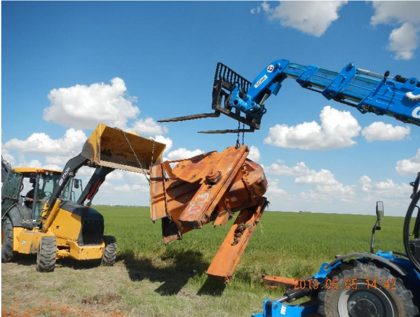
Photo 5: Picking up and relocating gear box for loading.
