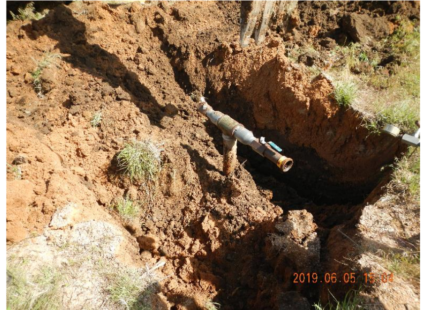
Photo 6: Excavating wellhead flow line.
