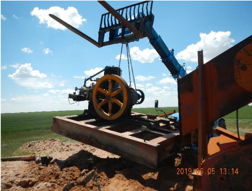
Photo 3: Removing prime mover and section of pumping unit base after being cut off.
