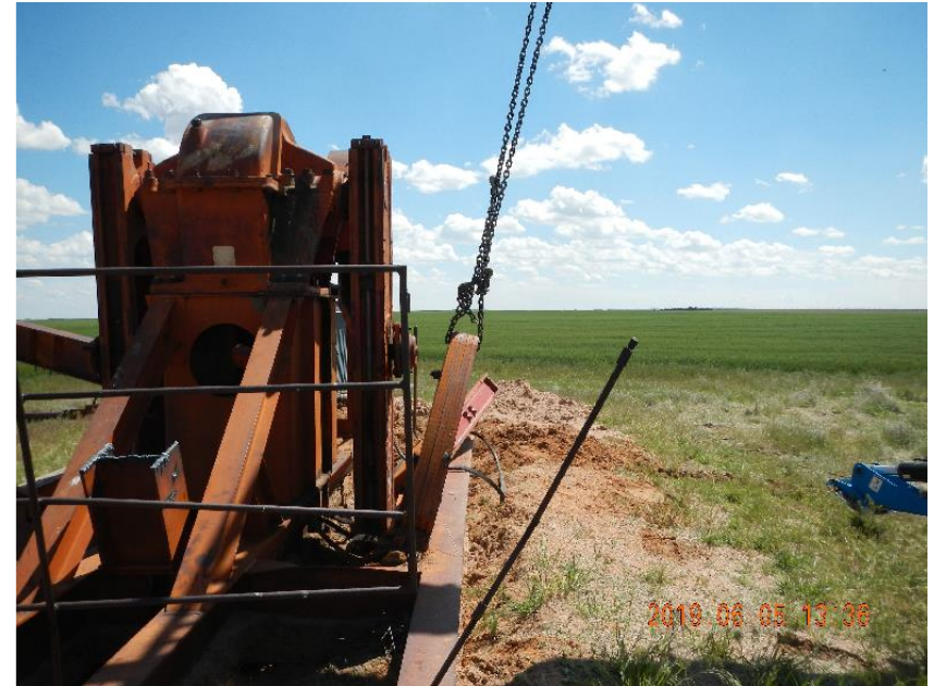
Photo 4: Removing counter weights.
