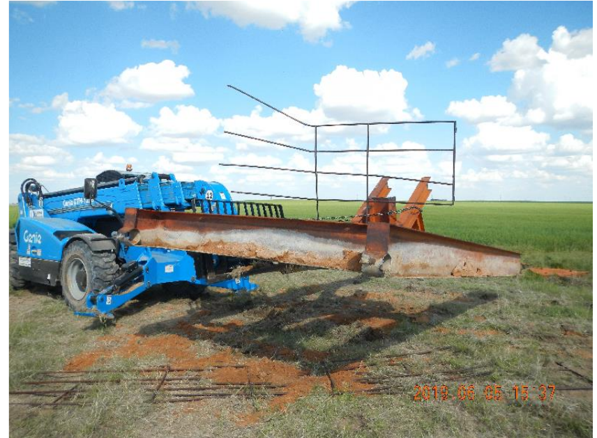
Photo 8: Relocating cut off section of pumping unit base.
