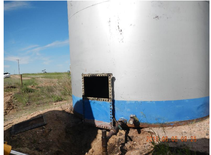
Photo 4: P3 entry top portion of entry hatch removed.
