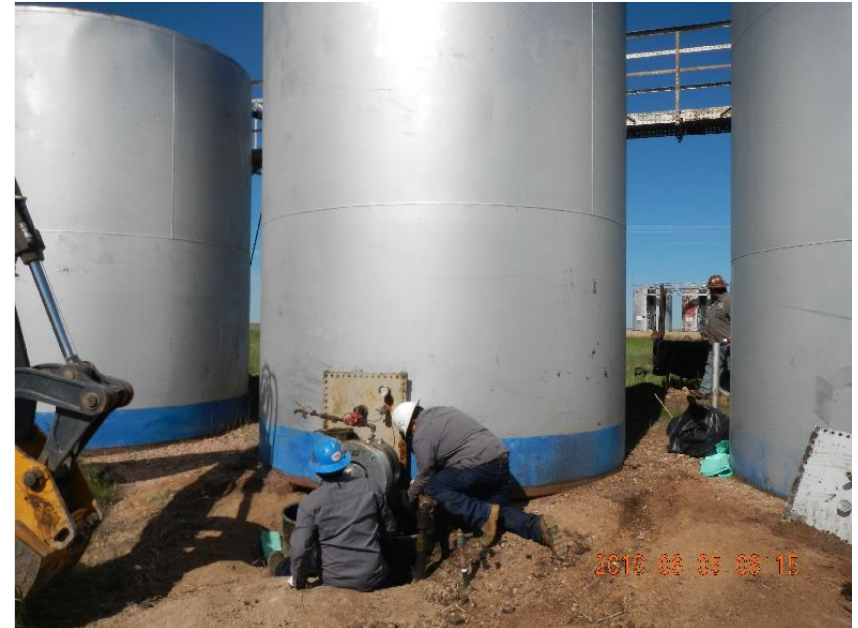
Photo 2: Removing entry hatch from P2.
