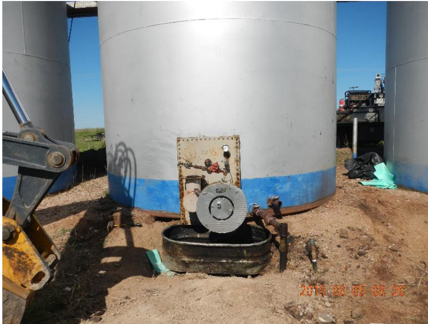
Photo 3: Excavated area below P2 entry hatch with trough installed to catch fluids.
