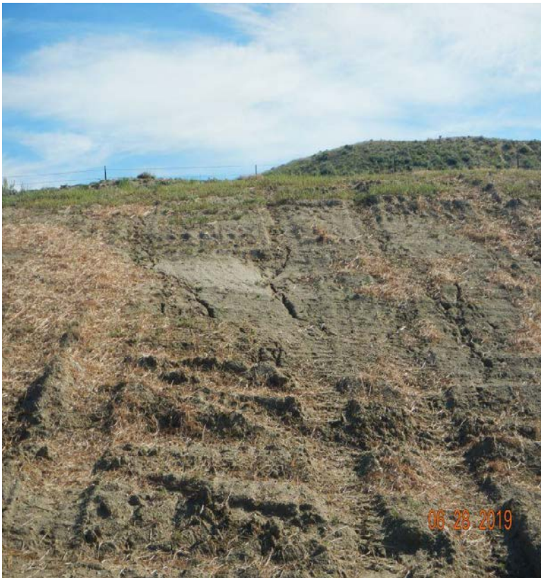
Photo#4: Area where erosion is commencing on North Cut slope.
