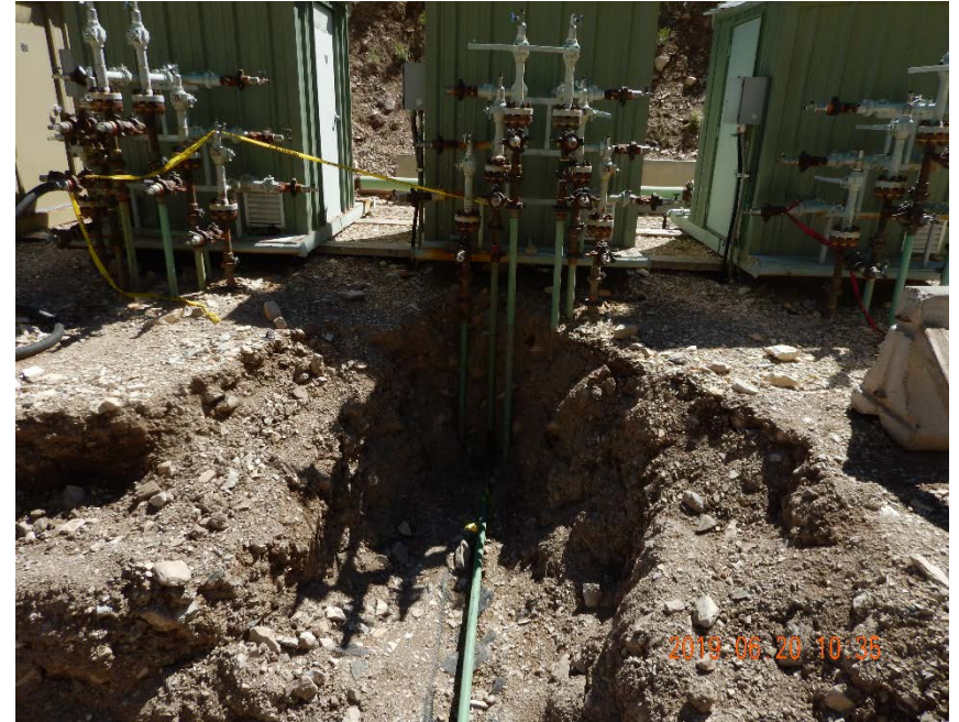
Photo #4 – Flowline equipment daylighting inside of excavation.
