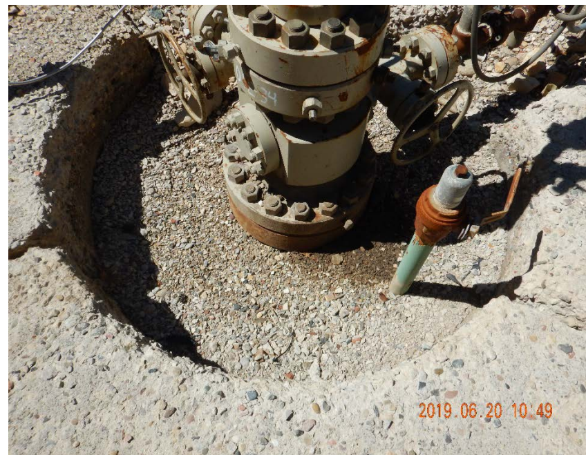
Photo #14 - NP EF01E-34 P27 595 wellhead with oil-stained material.
