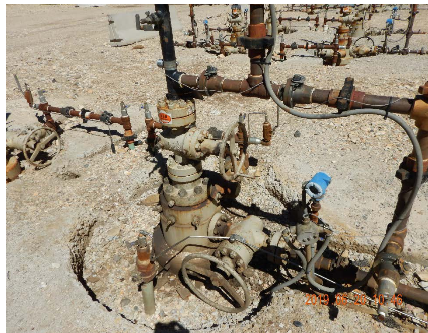
Photo #10 - NP EF01B 34 P27 595 wellhead with oil-stained material.
