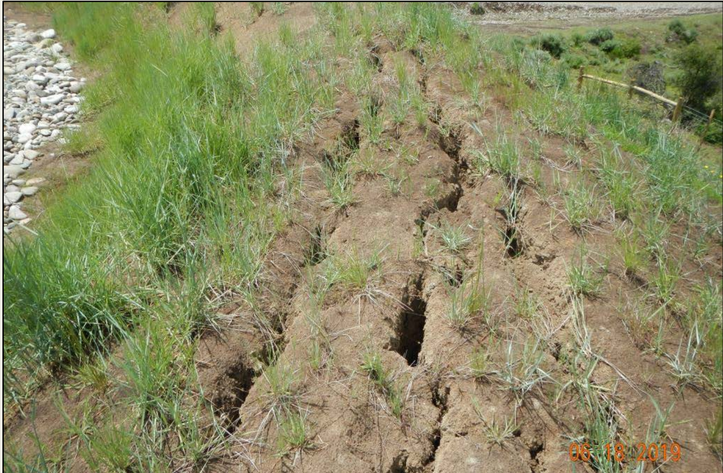
Photo 3. View of soil cracking up to 10 inches deep within the northern berm.
