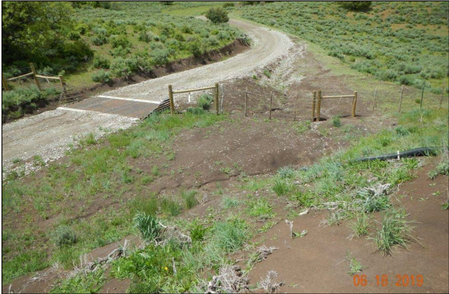
Photo 6. View of area in the northwestern project area where soils are not stabilized and erosion is occurring as stormwater flows north from the project area.
