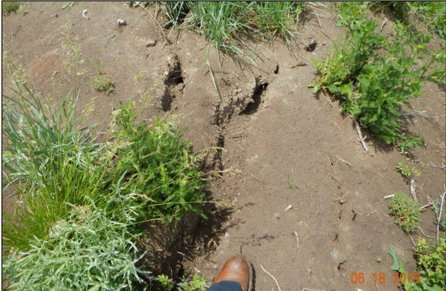
Photo 5. View of cracking within the eastern well pad berm.
