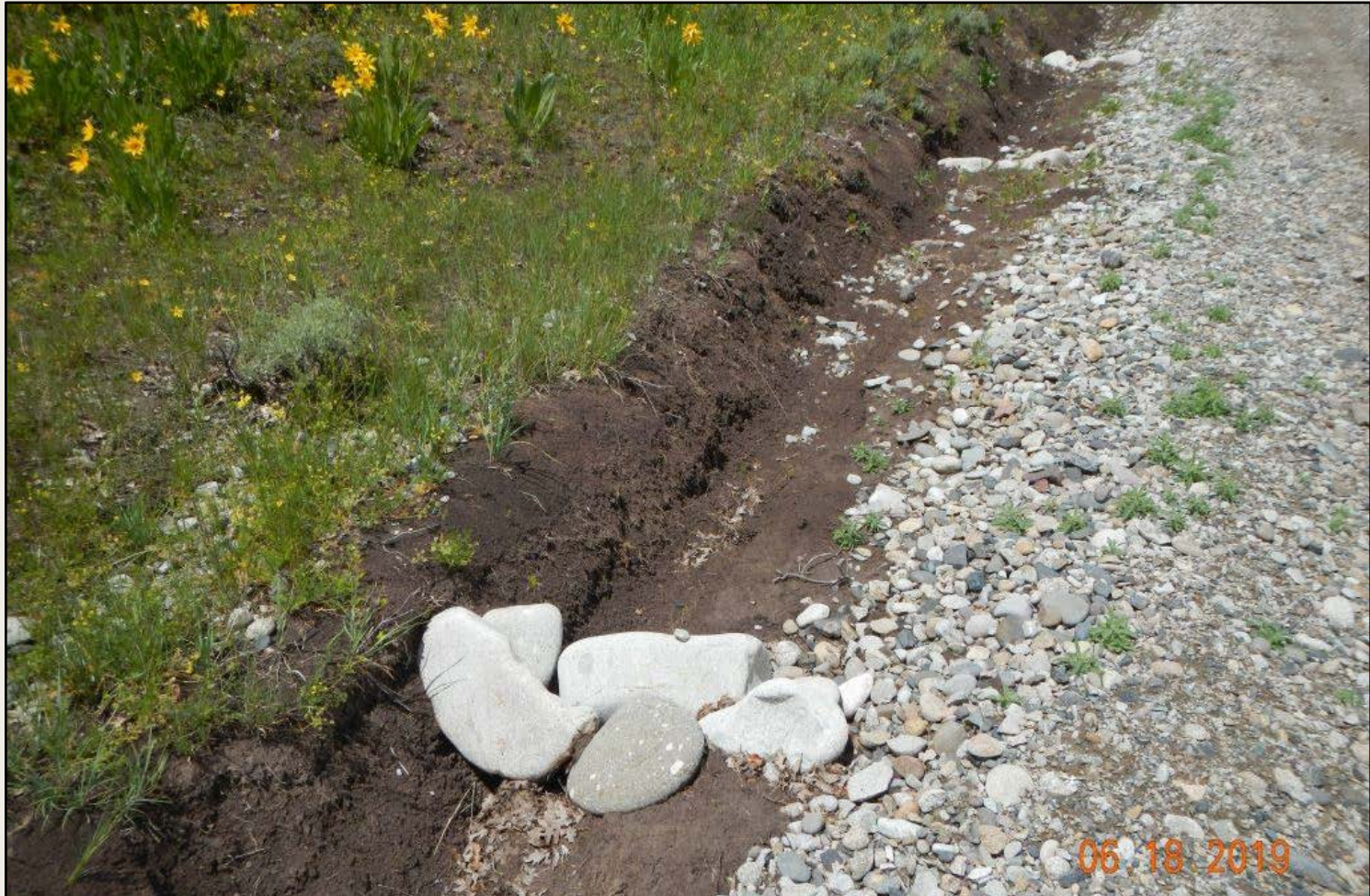
Photo 7. View of cobble velocity checks along the northwestern access road. These are not sufficient as erosional down-cutting from high velocity flows, and sediment deposition where flows settle, is evident.
