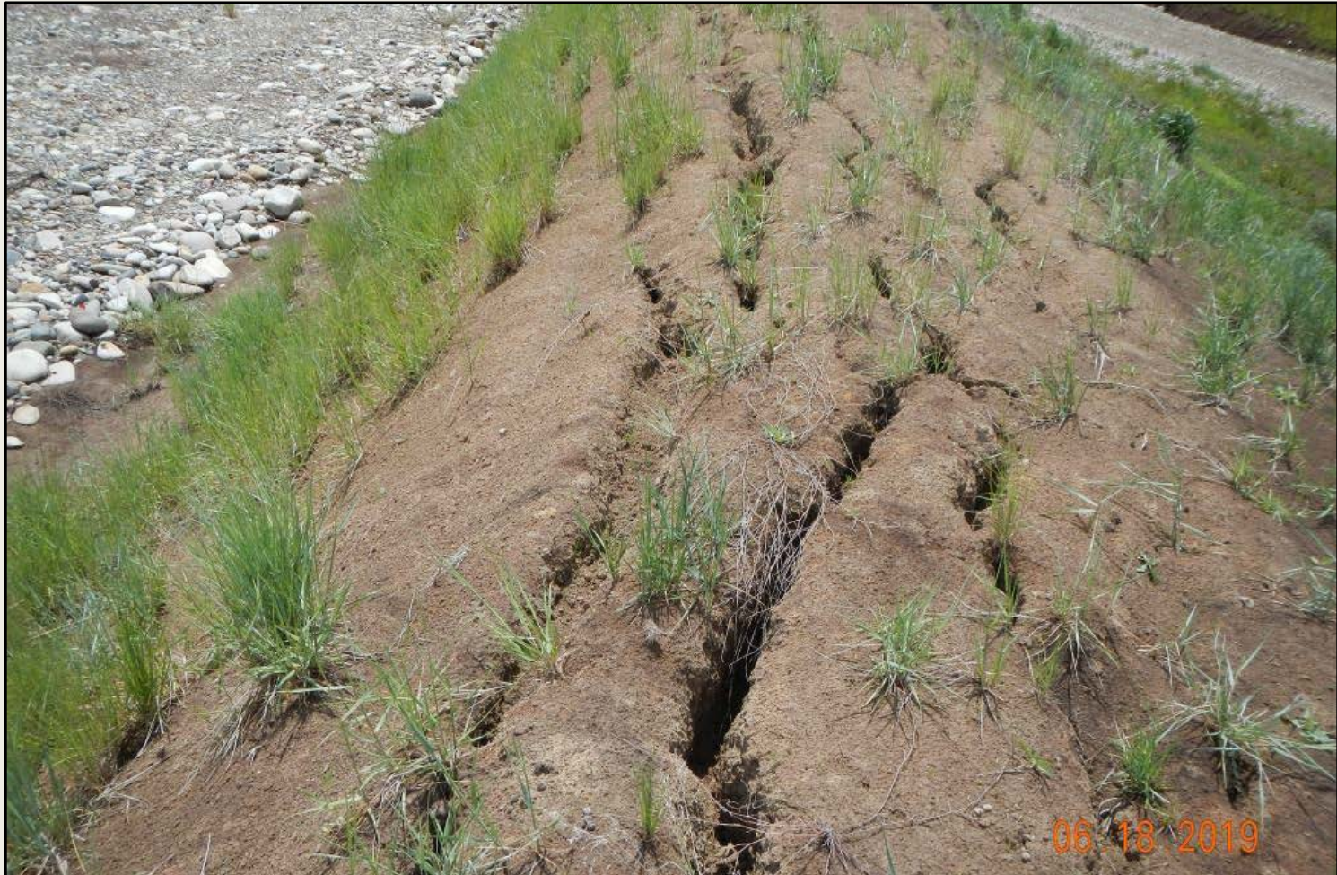
Photo 4. View of more soil cracking within the well pad berm.
