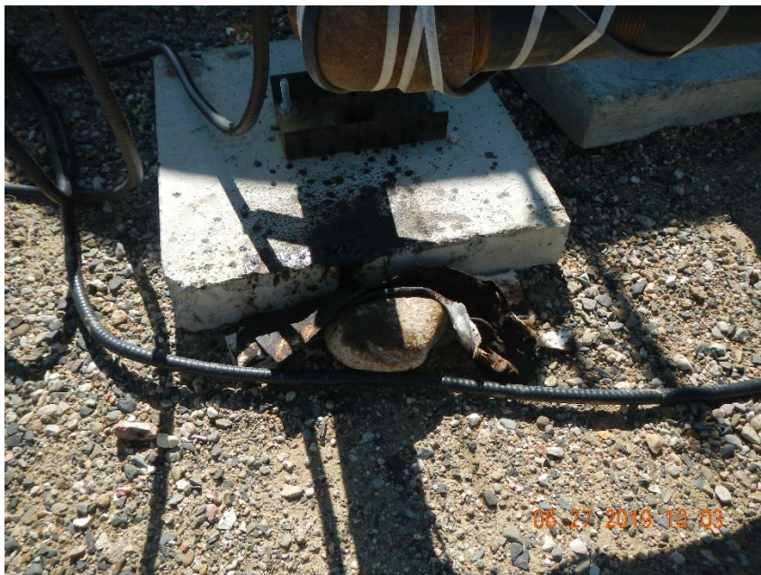
Photo 5. Drip at separator with rag held in place with rock beneath drip.
