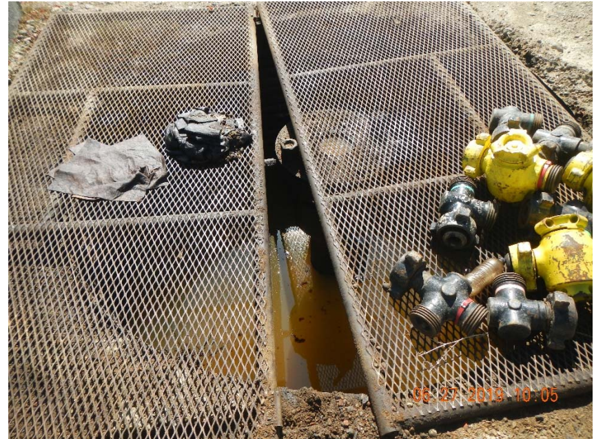
Photo 10. Trash and debris, stormwater with a sheen in cellar.
