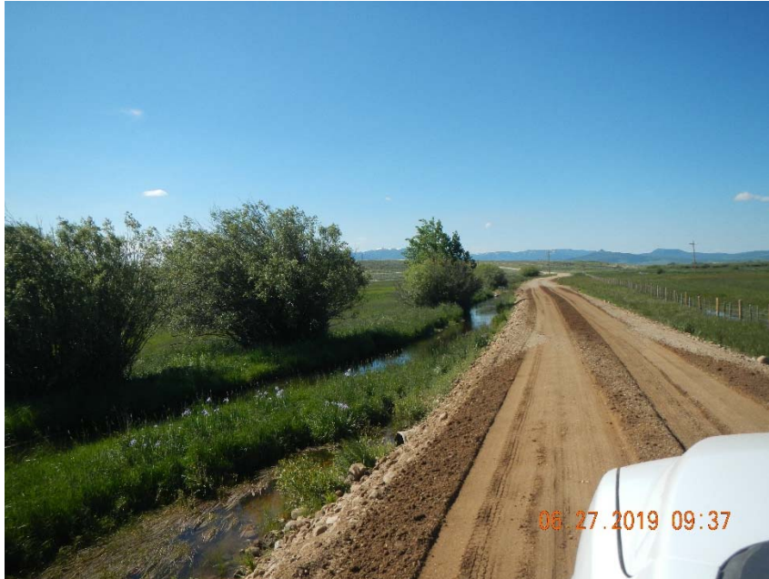
Photo 1. Access road with fresh material and no stormwater BMPs.
