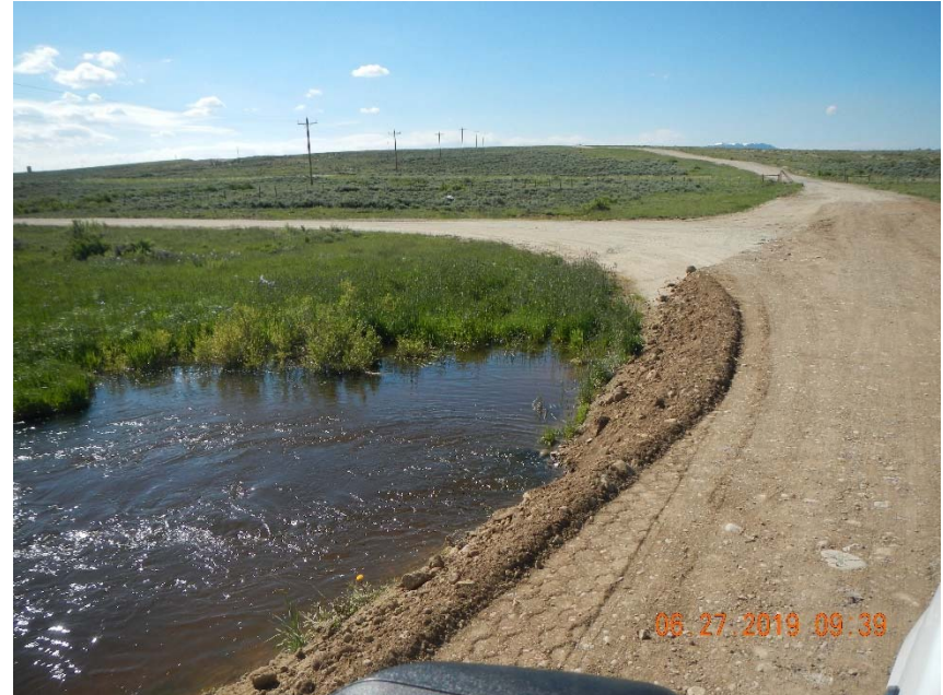
Photo 2. Access road with fresh material and no stormwater BMPs.
