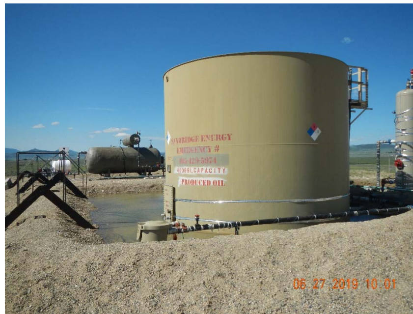
Photo 4. Condensate tank labeled as crude oil.
