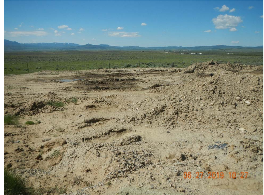
Photo 14. Perimeter berm on southeast corner of location has been compromised.
