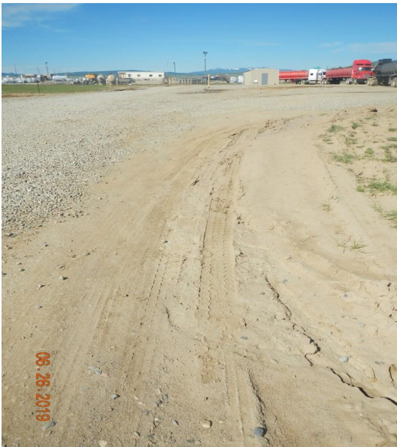
Photo#2: Showing results of lack of BMPs on Access Road.
