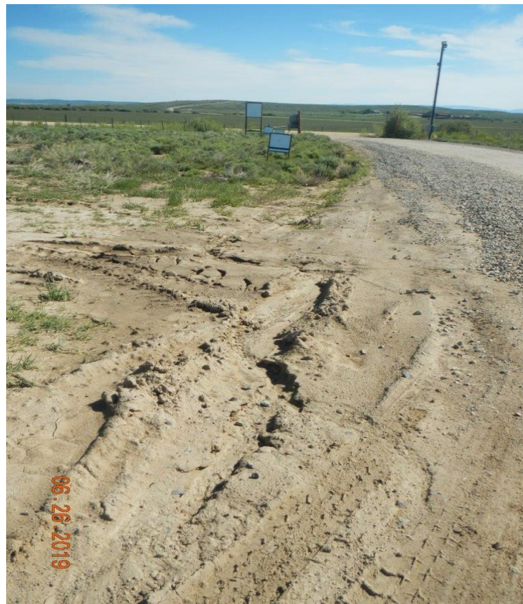
Photo#3: Showing results of lack of BMPs on Access Road.
