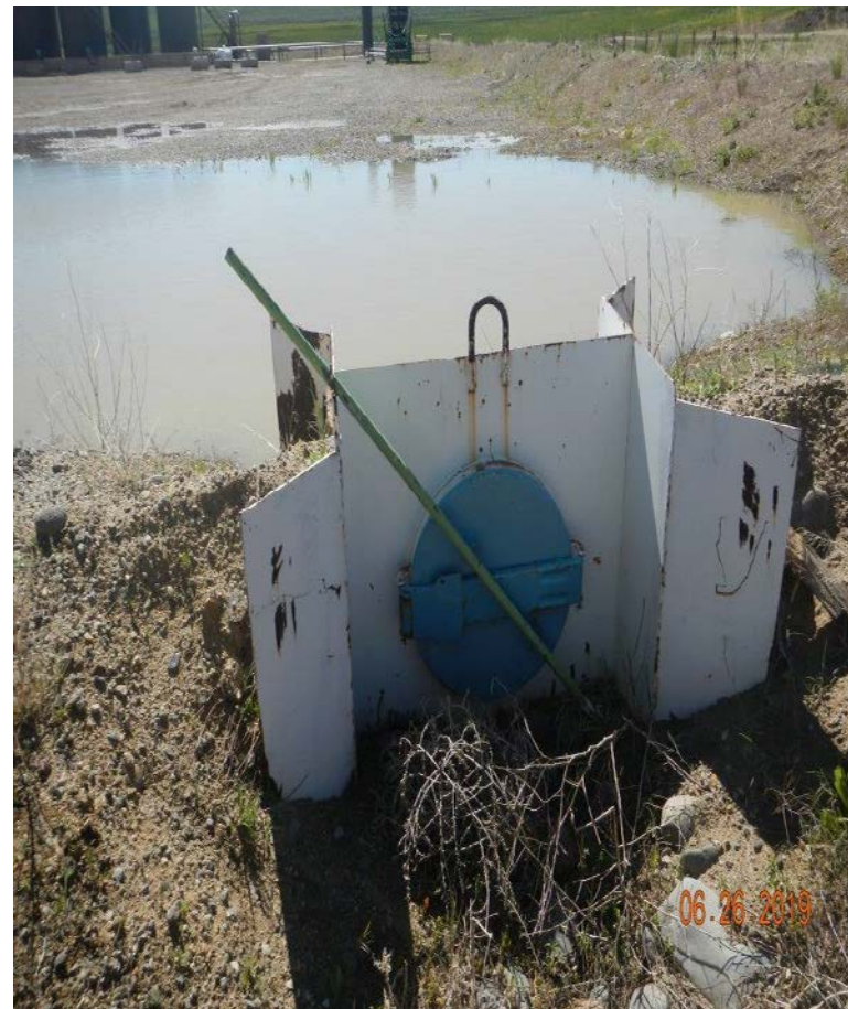
Photo#5: Weir installation at SW corner, looking into pad.
