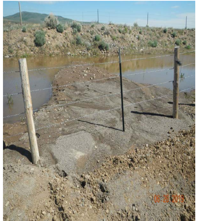
Photo#3: Sediment deposit that occurred when corner washed out.
