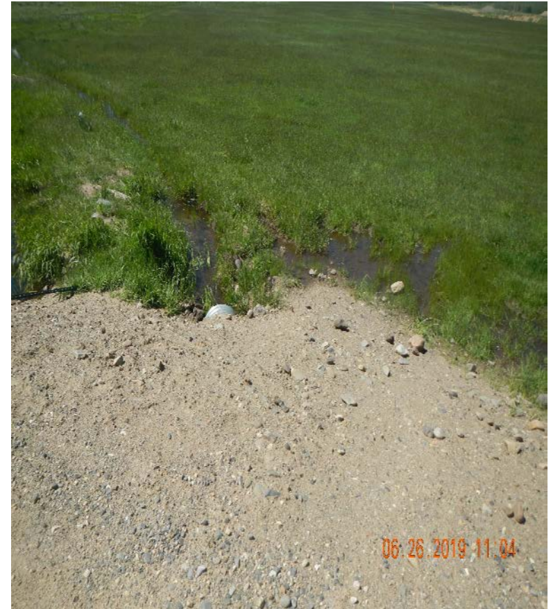
Photo#9: Lack of BMPs along access road at culvert.
