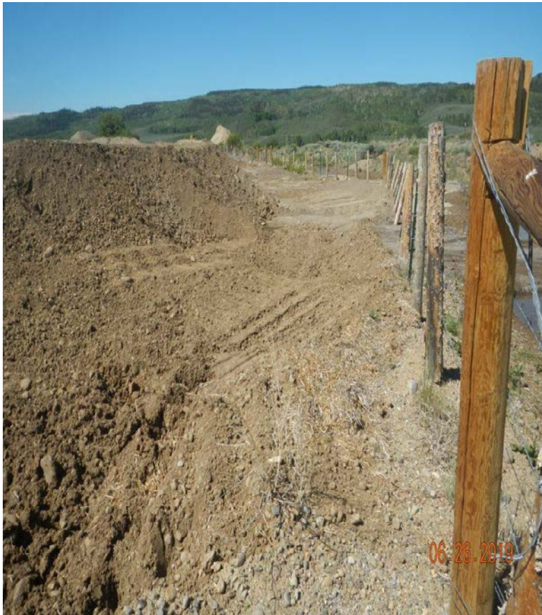
Photo#2: NW Corner of site, repaired, where washout occurred.
