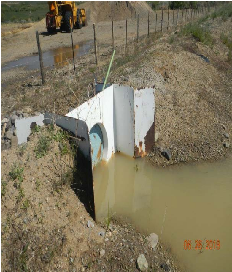
Photo#4: Weir installation at SW corner, looking out to perimeter.
