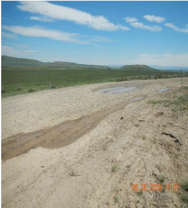
Photo#8: Lack of BMPs along both sides of access road.
