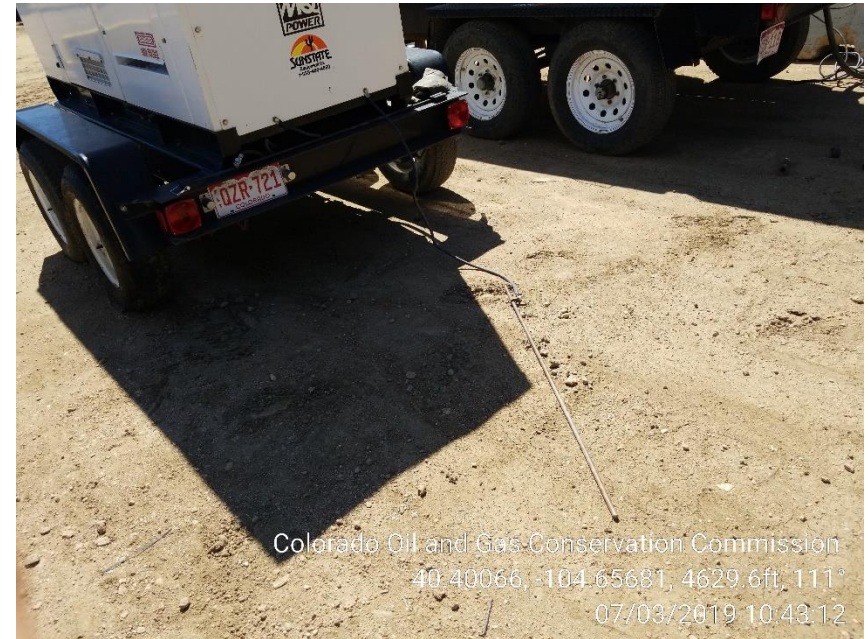
Photo 2 – Generator not grounded, Crew working on getting it grounded today.
