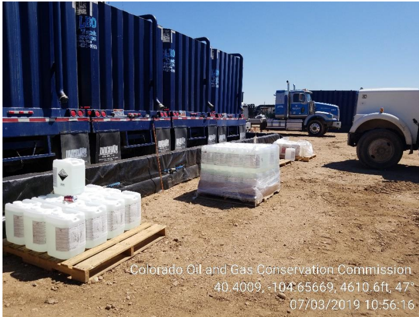
Photo 3 – Chemical not in secondary containment, crew working on getting containment and covered
