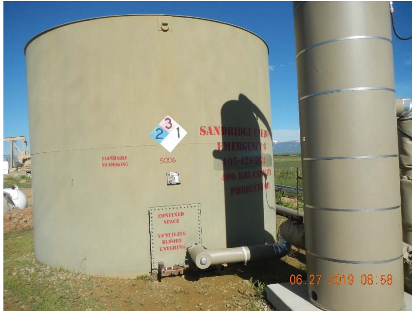
Photo 7. Condensate tank labeled as crude oil. No liner apparent, berm not compacted.
