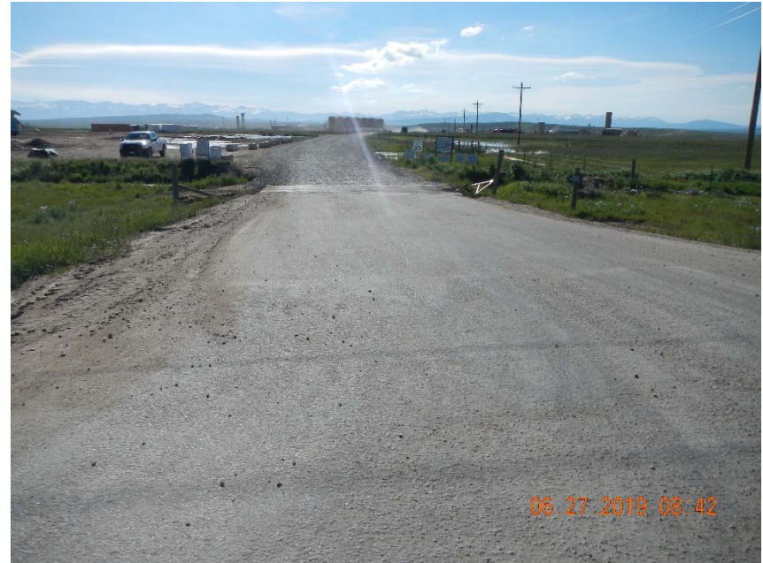
Photo 10. No tracking BMPs apparent at location entrance from highway.
