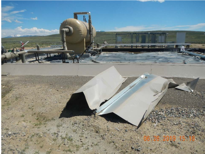
Photo 1. Containment parts becoming debris, unused equipment on location.
