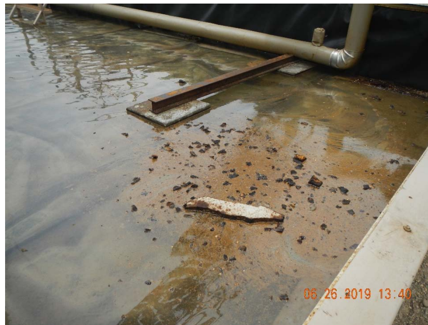
Photo 6. Free product on stormwater in metal berm.
