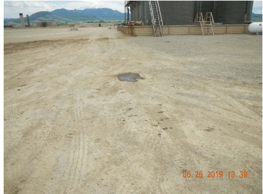
Photo 4. Example of stained soil on location.
