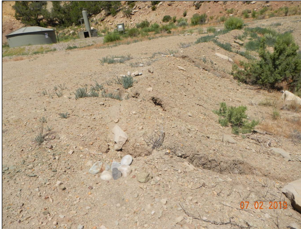
Photo #11 Storm Water Erosion moving off location on East side of location
