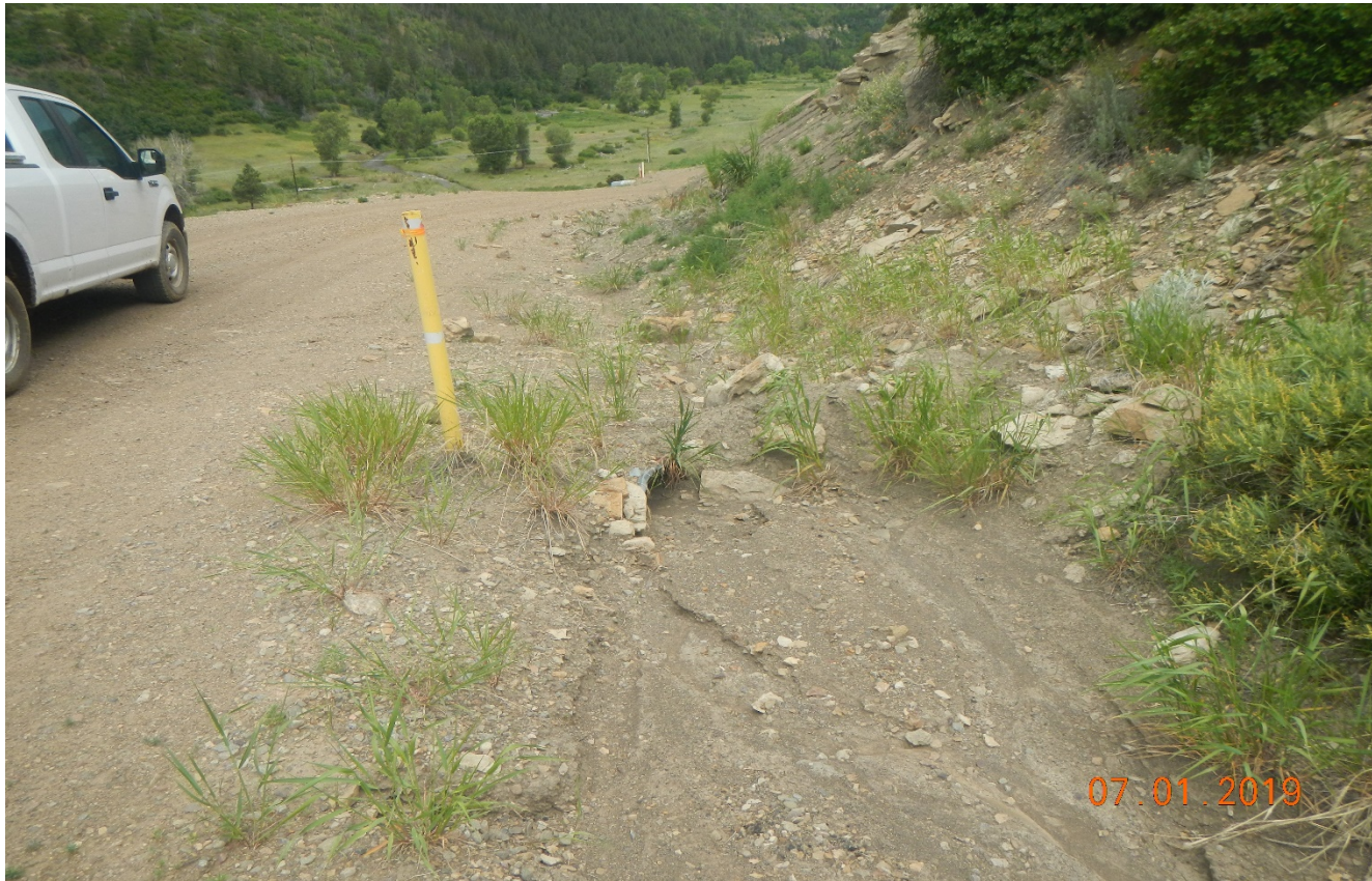
Photo 1. The culvert is full of sediment along the access road.
