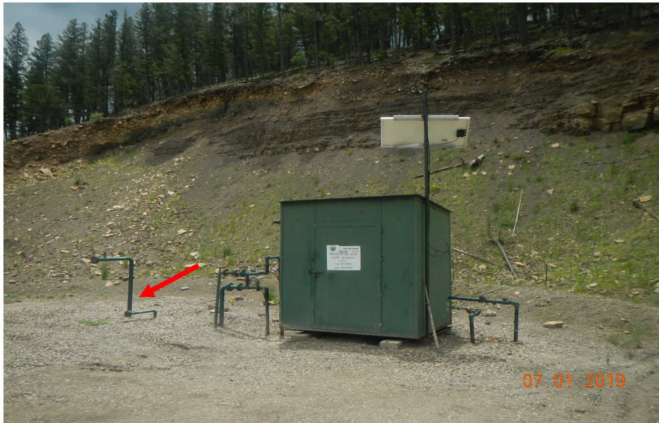
Photo 2. Facing toward the location. Unused risers not LO/TO.
