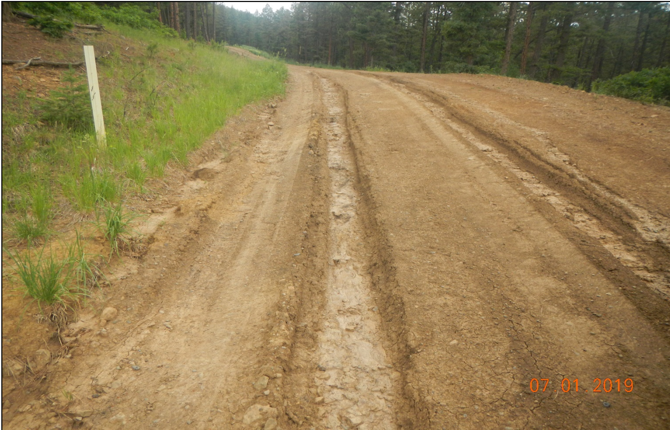
Photo 2. Vehicle ruts remain along the road which is a conveyance for stormwater erosion.
