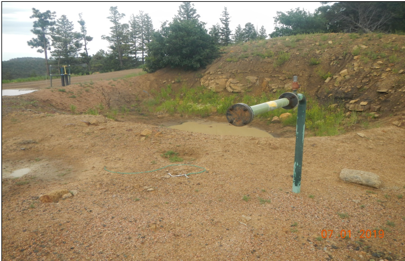
Photo 6. Pipe risers with not LO/TO are unused equipment.
