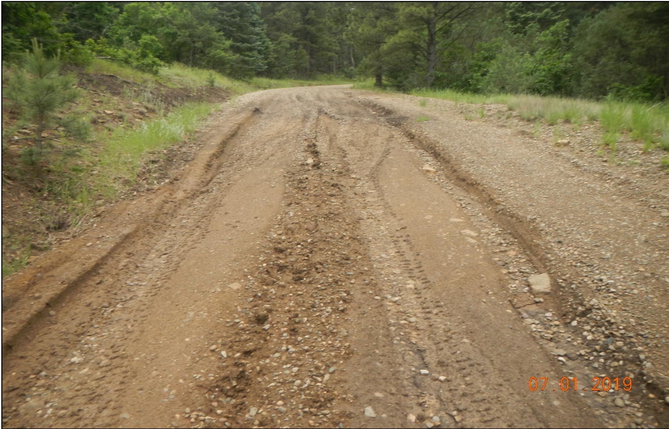
Photo 1. Vehicle ruts remain along the road which is a conveyance for stormwater erosion.
