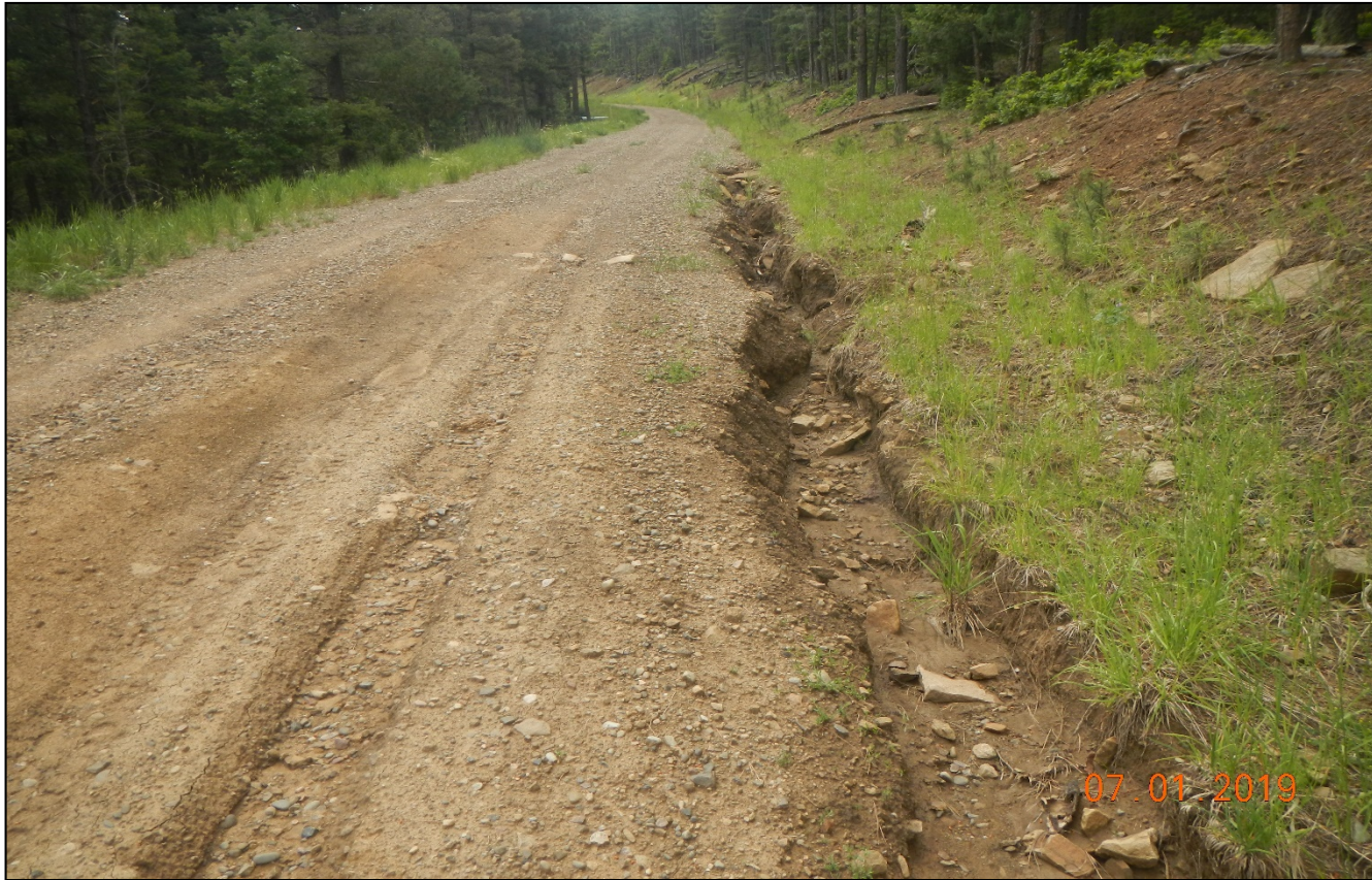
Photo 3. There is erosion occurring along the side of the road. No BMP's present.
