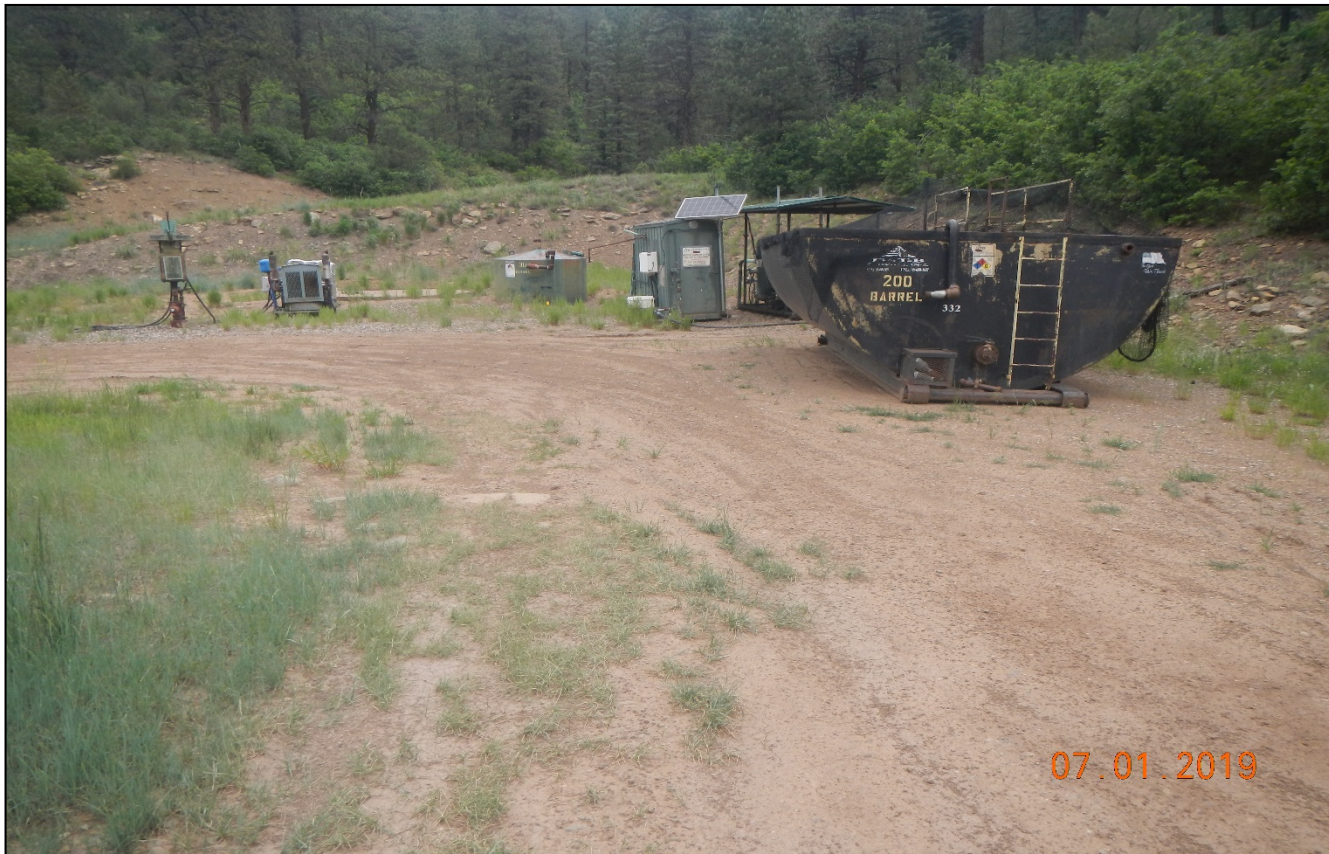
Photo 3. Facing toward the well site. There is no secondary containment around produced water tank.
