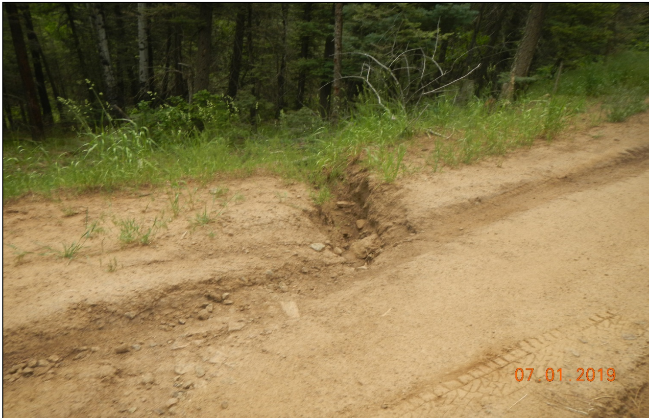
Photo 2. Stormwater flowing across the road shown in the previous photo has not been repaired.
