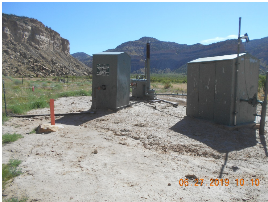
Separator and Meter housings.
