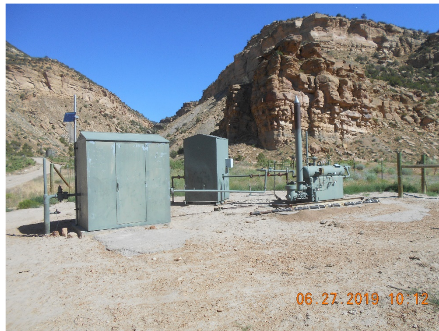
Separator and Meter housings. Junk pipe around separator needs removal.
