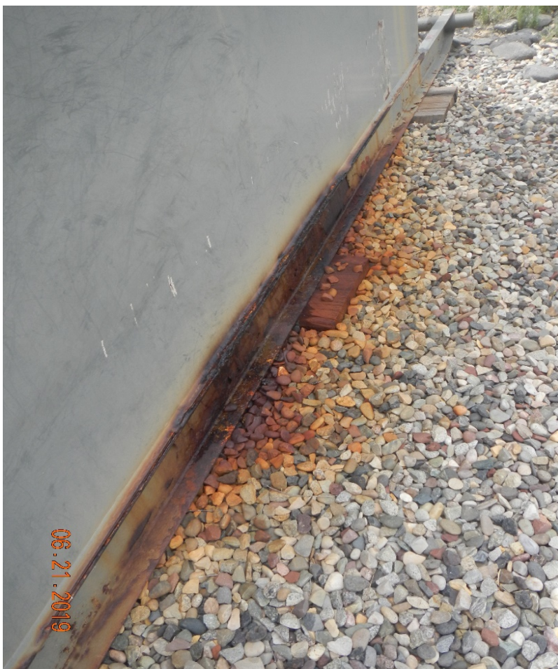
Photo#4: Repair of leak has failed.
