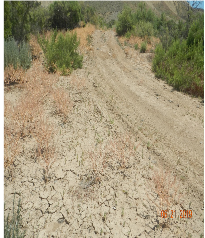
Photo#5: Access road does not have adequate Stormwater controls.
