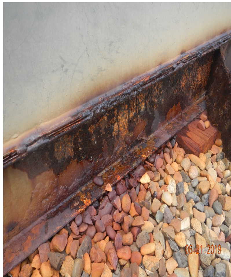
Photo#5: Repair of leak has failed.
