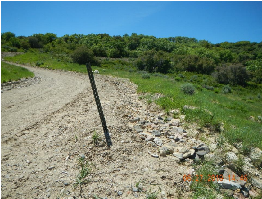
Sediment build up in ditch going into checkdam.
