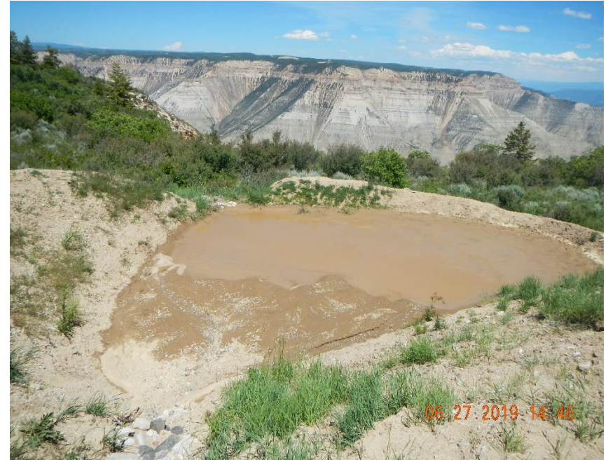
Sediment build up in checkdam.
