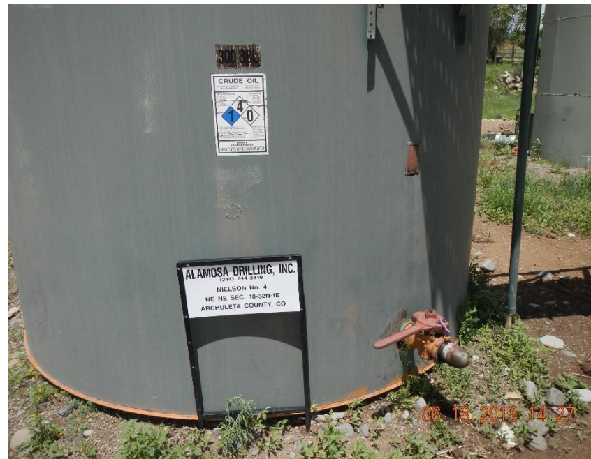
Nielson #4 300 bbl. AST. Tamper evident seal on load out valve handle.
