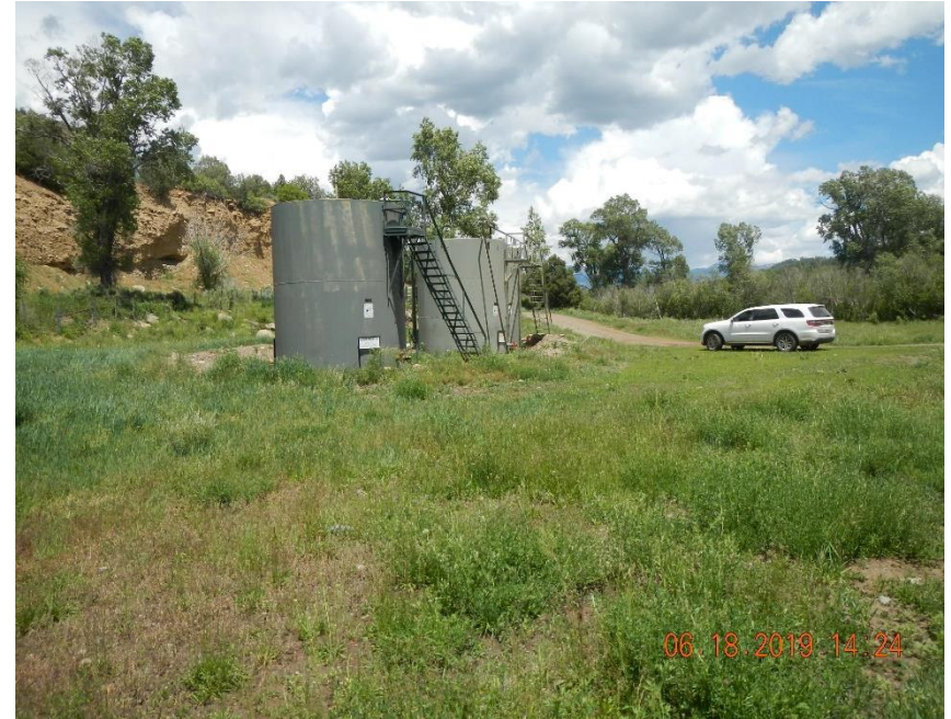
Nielson #4 tank battery. Secondary containment berm shared with Albert Martinez #1 ASTs.
