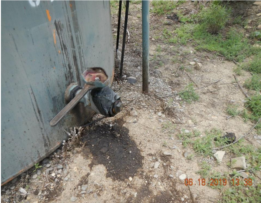
Stained soil beneath load out valve.
