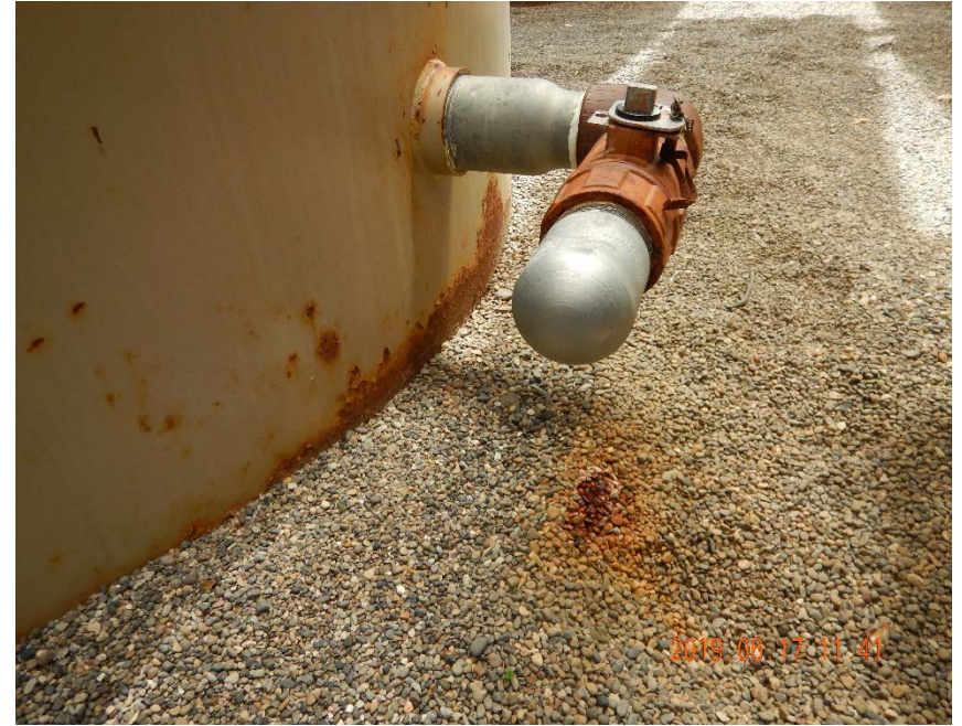
Photo #10 – Accumulation of salt and rust observed beneath bullplug attached to Tank ID #114027.
