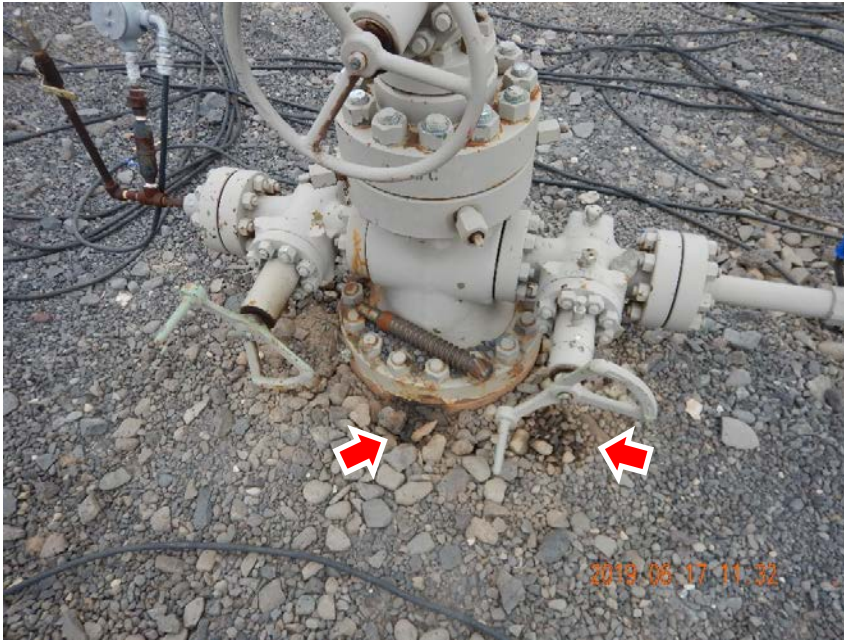
Photo #5 – McDaniel 2-16C wellhead. Note accumulations of oil-stained soil observed at wellhead (red arrows). Well sign was down on inspection date.
