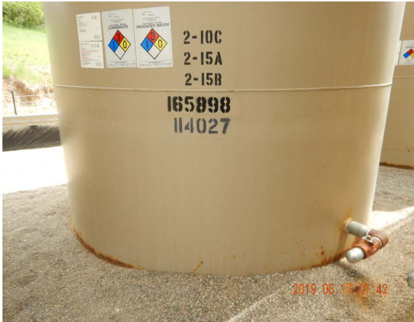
Photo #9 – Tank ID #114027. Accumulation of rust and salt observed beneath bullplug (next photo).
