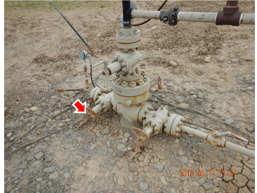
Photo #4 – McDaniel 2-10 wellhead. Note an audible gas leak was observed from this wellhead on inspection date (red arrow depicts approximate leak location). Operator was notified of leak via phone on inspection date.
