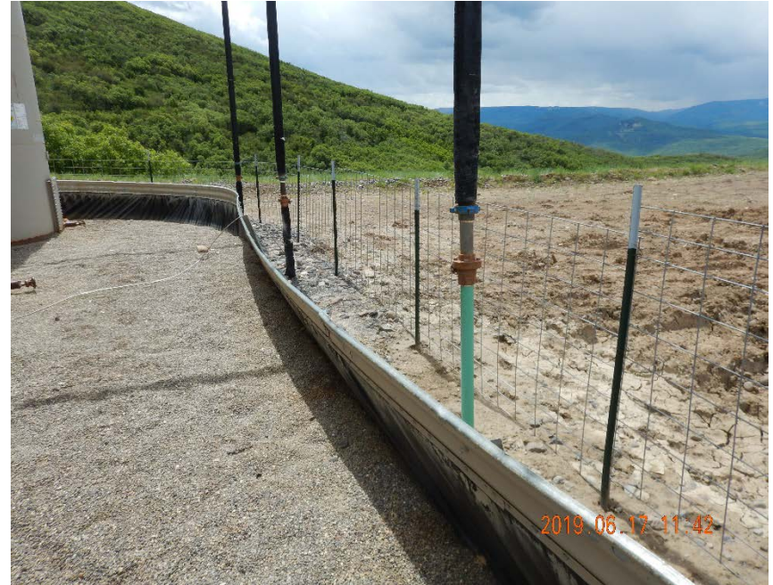
Photo #8 – Bent section of tank battery berm (south side).
